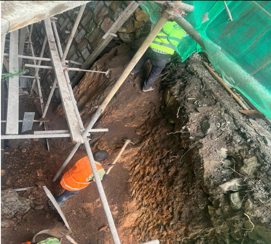
Phase 4: Retaining wall excavation remained portion
