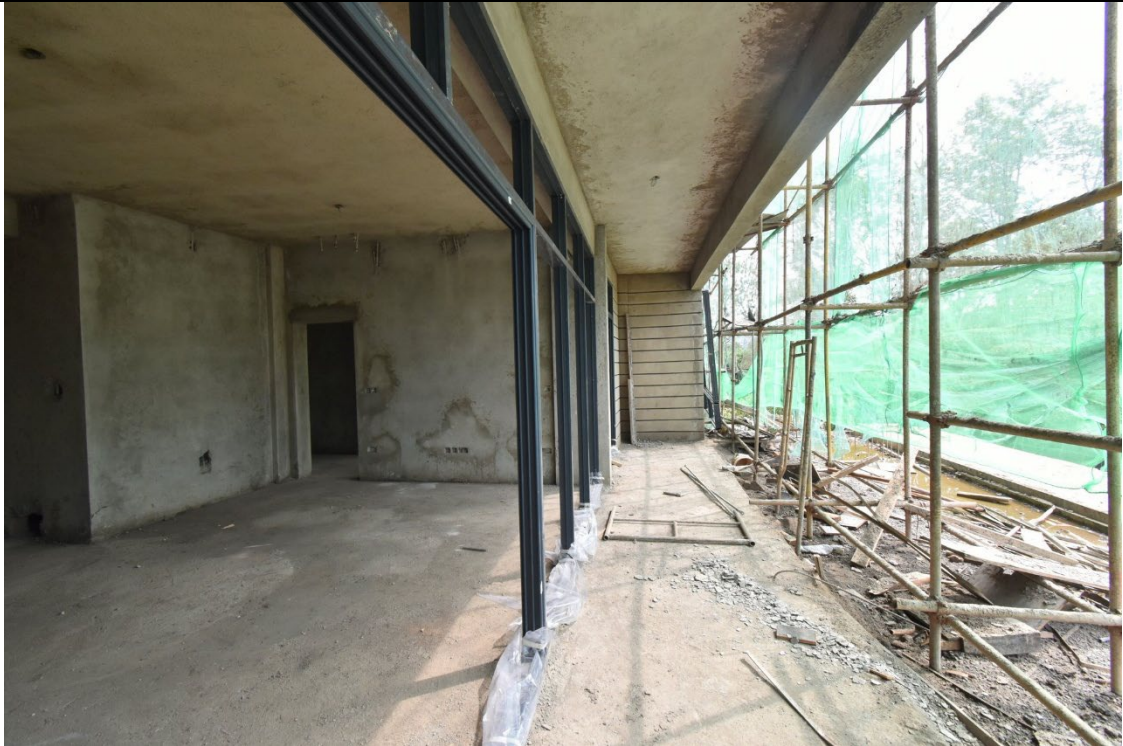
One of the apartments on the first floor, showing curtain wall aluminium
