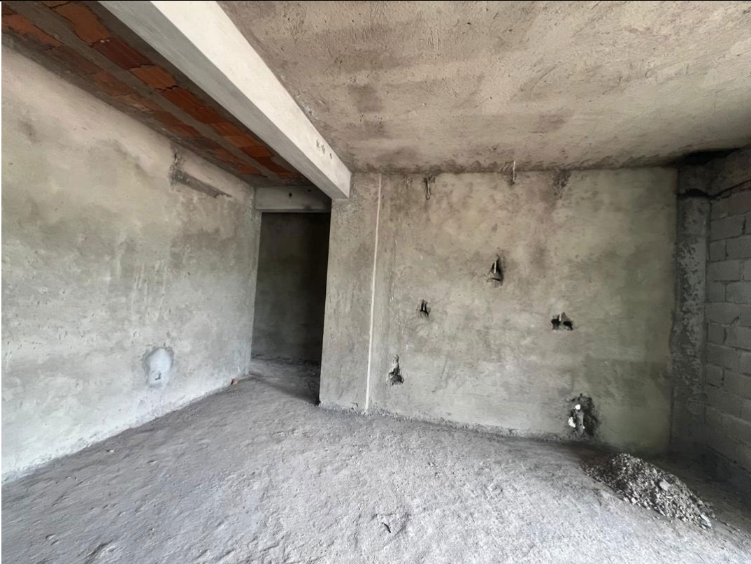
Internal walling in progress level 2&3
