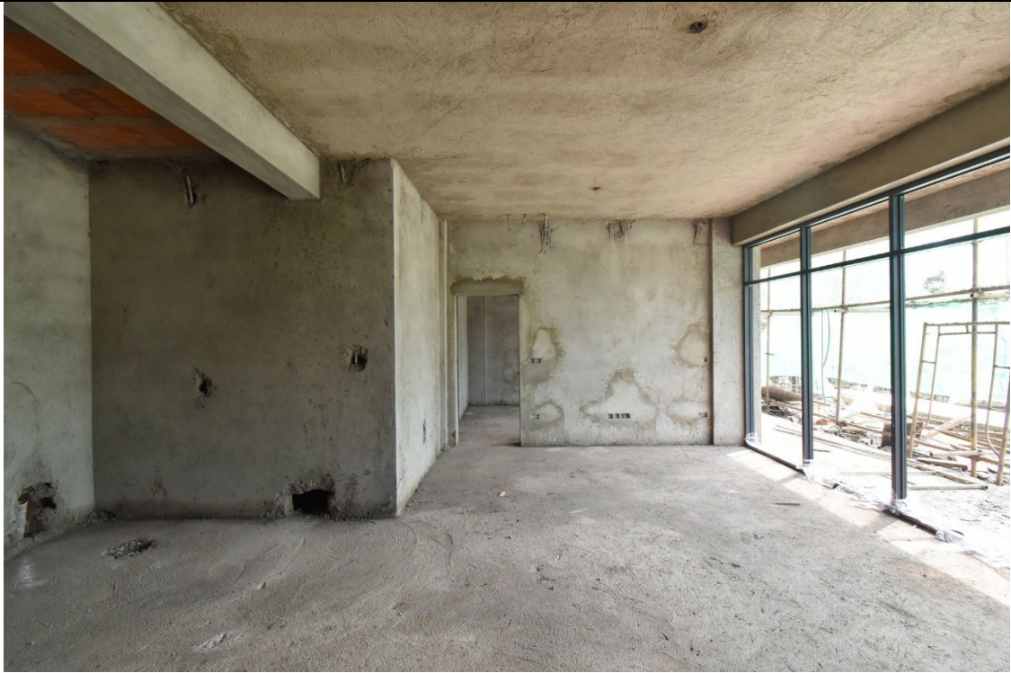
Internal walling in progress level 2&3, with curtain wall works
