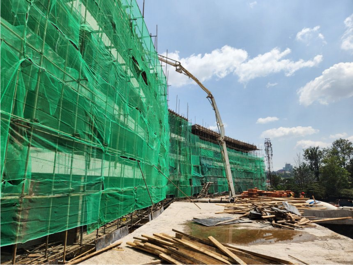
View of Phase 3 & 4 casting and pool area
