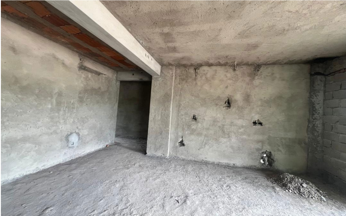
Phase 3&4 :Internal walling in progress level 2&3
