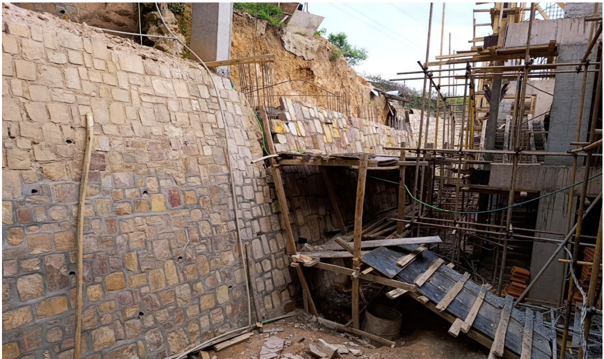
Phase 3 works showing: Masonry walling of retaining wall
