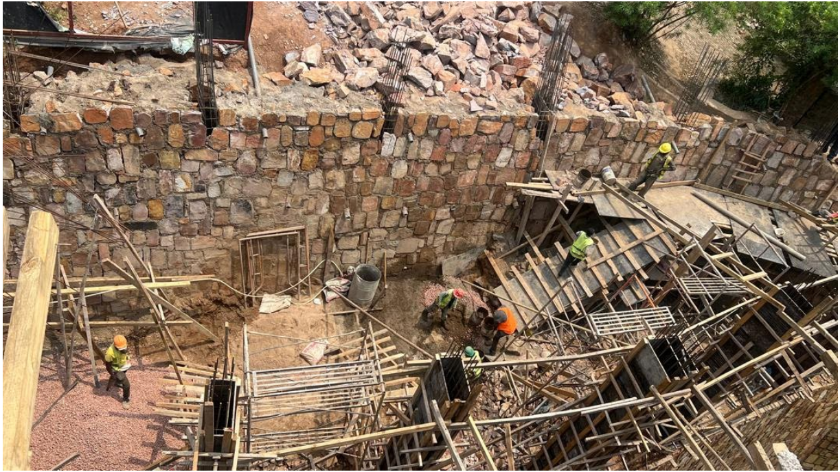
Retaining wall progress at phase 3 upper ground
