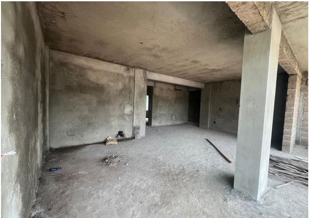
Phase 3&4 : Internal walling in progress level 2&3
