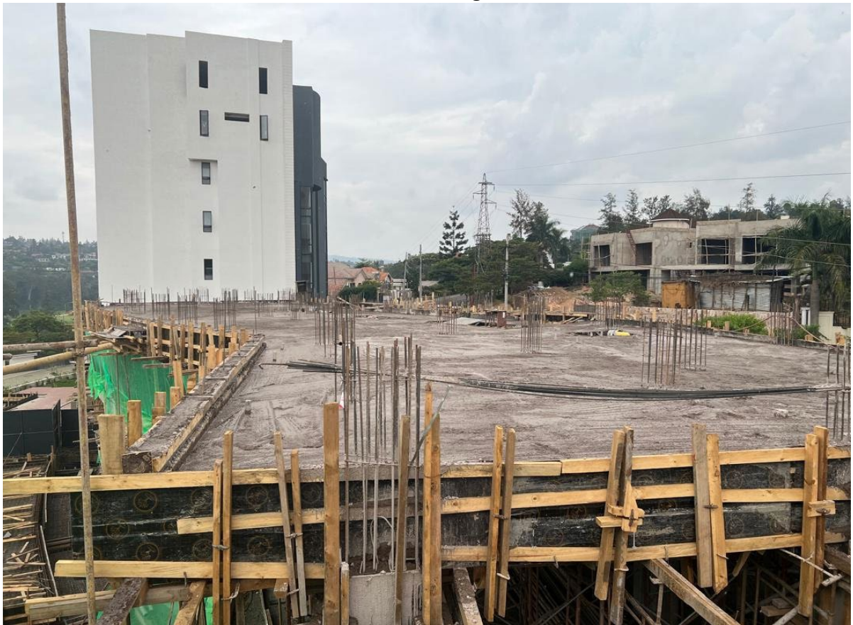
Phase 3 works showing: Concrete casting at level 6
