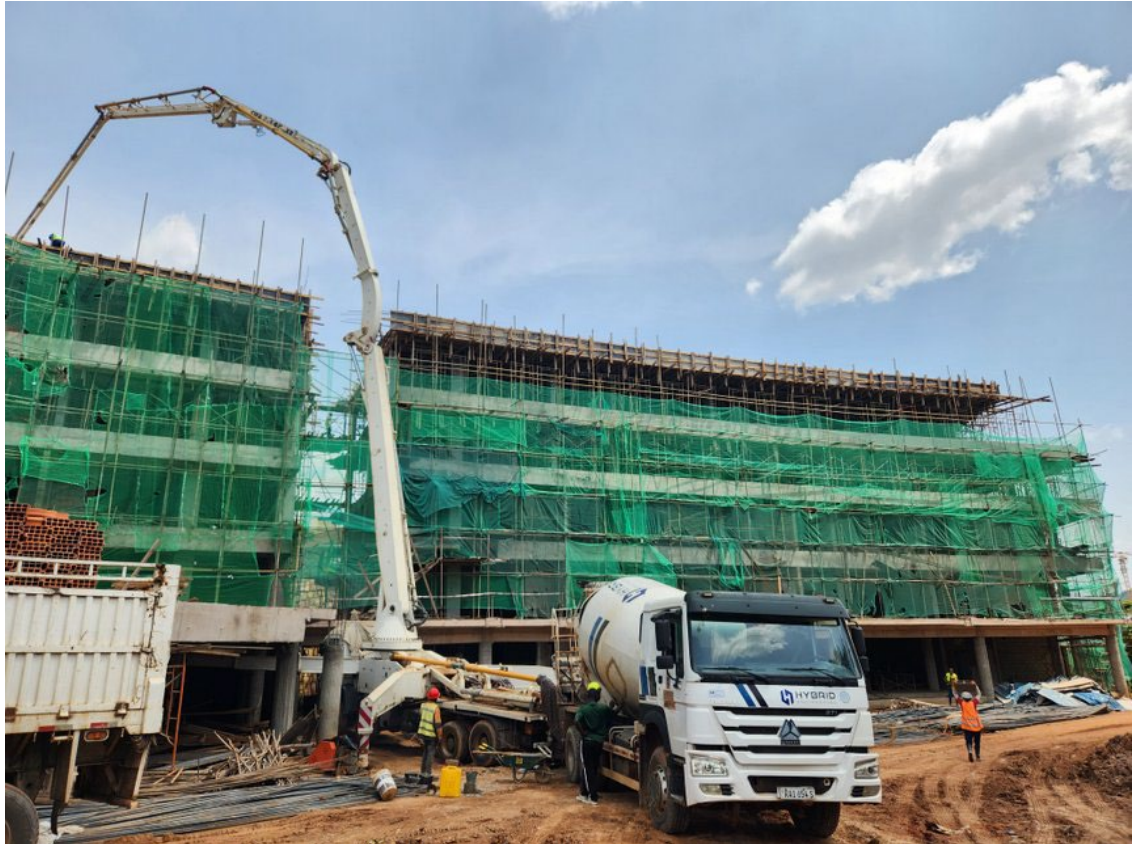
View of Phase 3 & 4 casting
