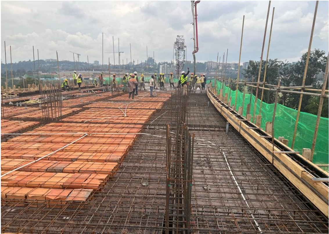
Phase 3/4 Slab casting Lv.6
