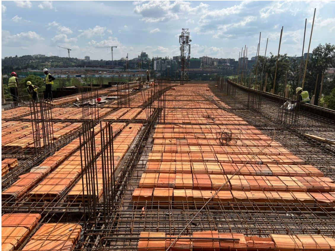
Phase 3/4 works showing: Formwork & steel reinforcement for slab on Lv. 5
