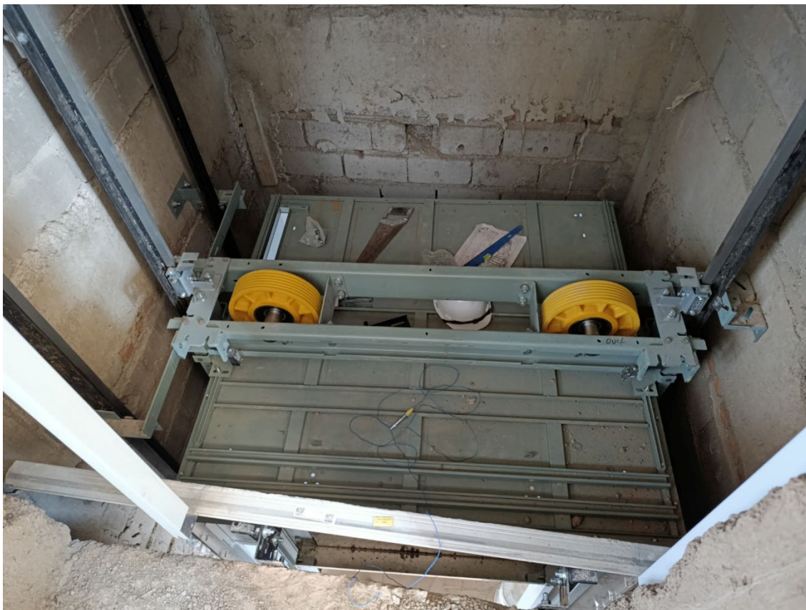
Phase 2 works showing: Installed lift car in the lift shaft
