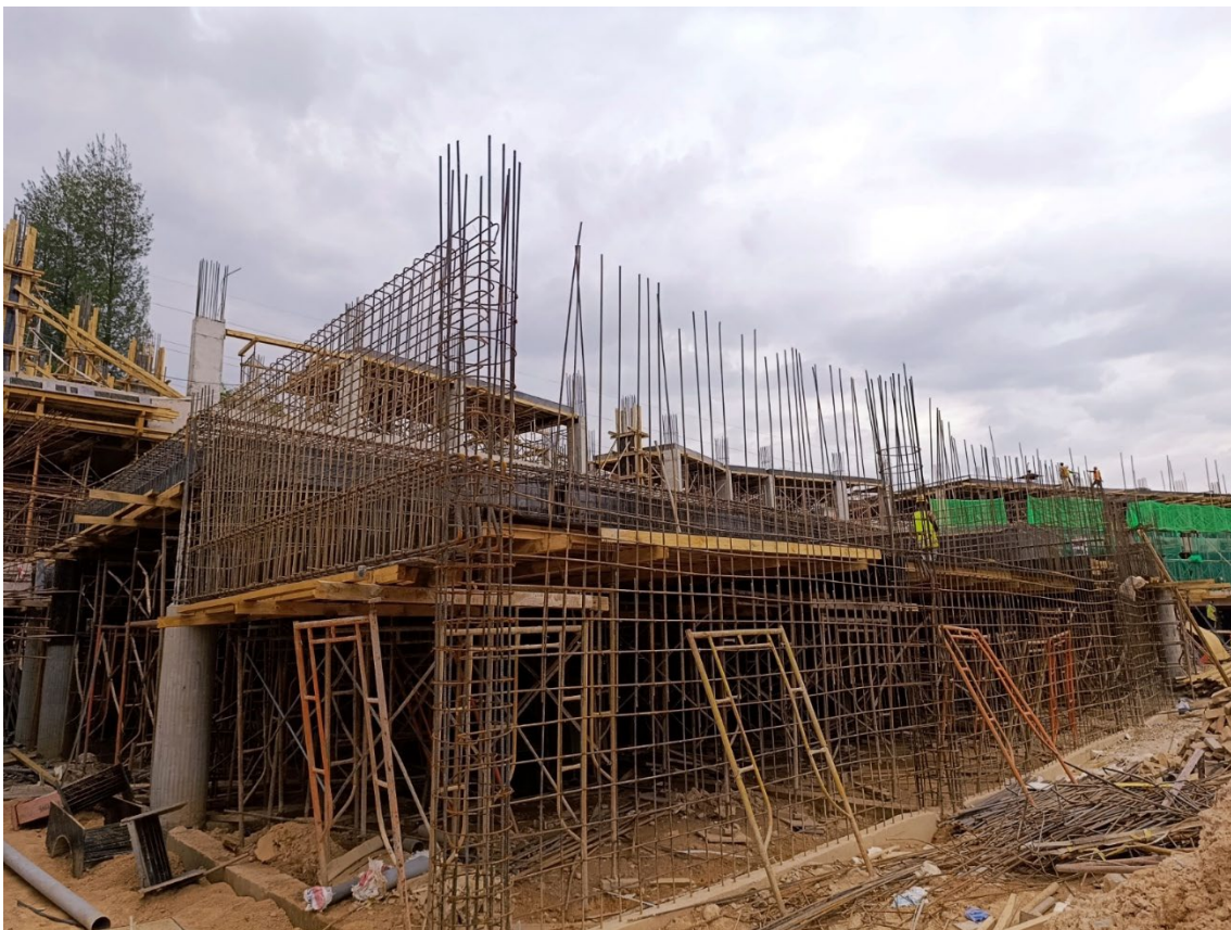
Phase 3 works showing: Steel work for pool & deck slab
