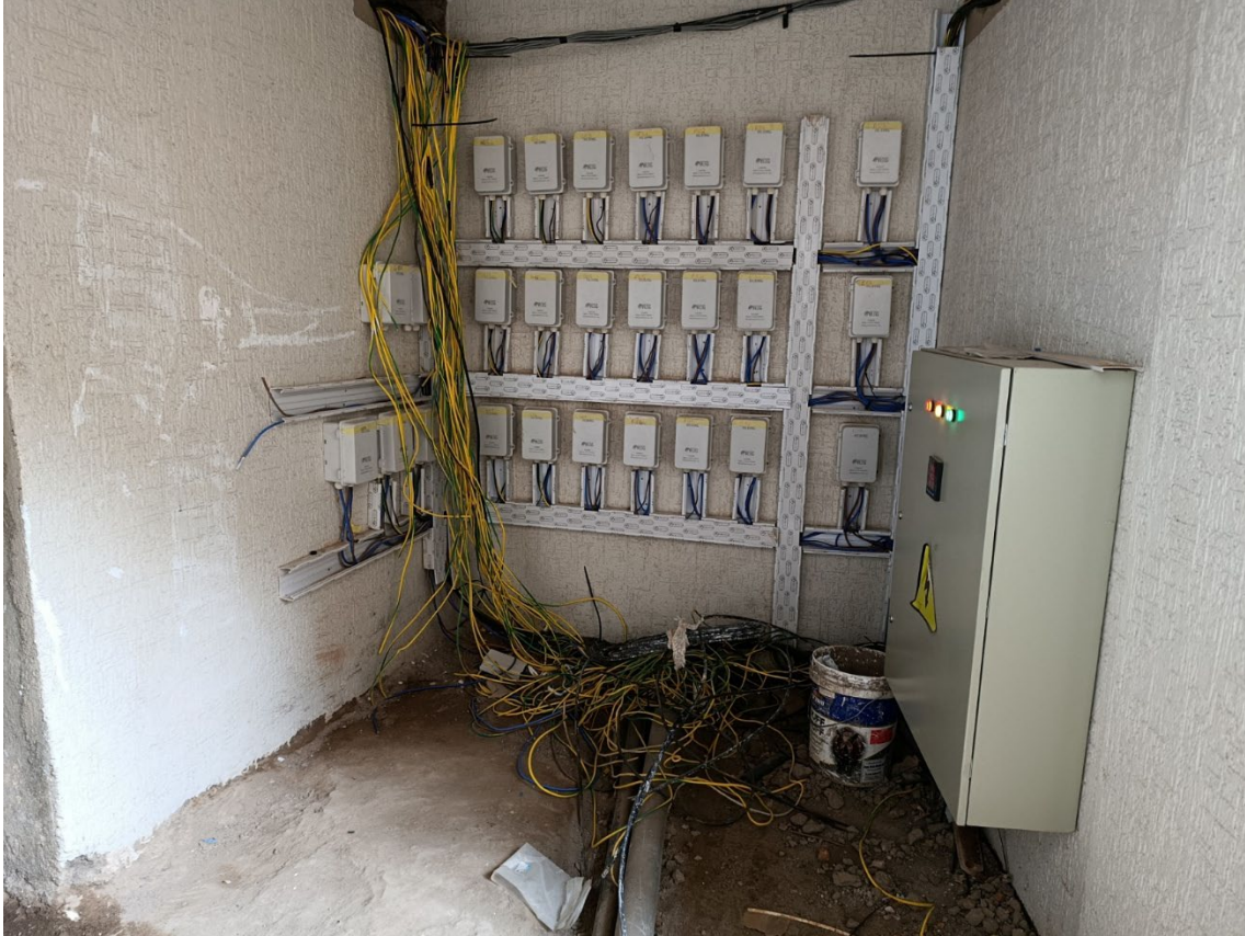
Phase 2 works showing: REG meters installed
