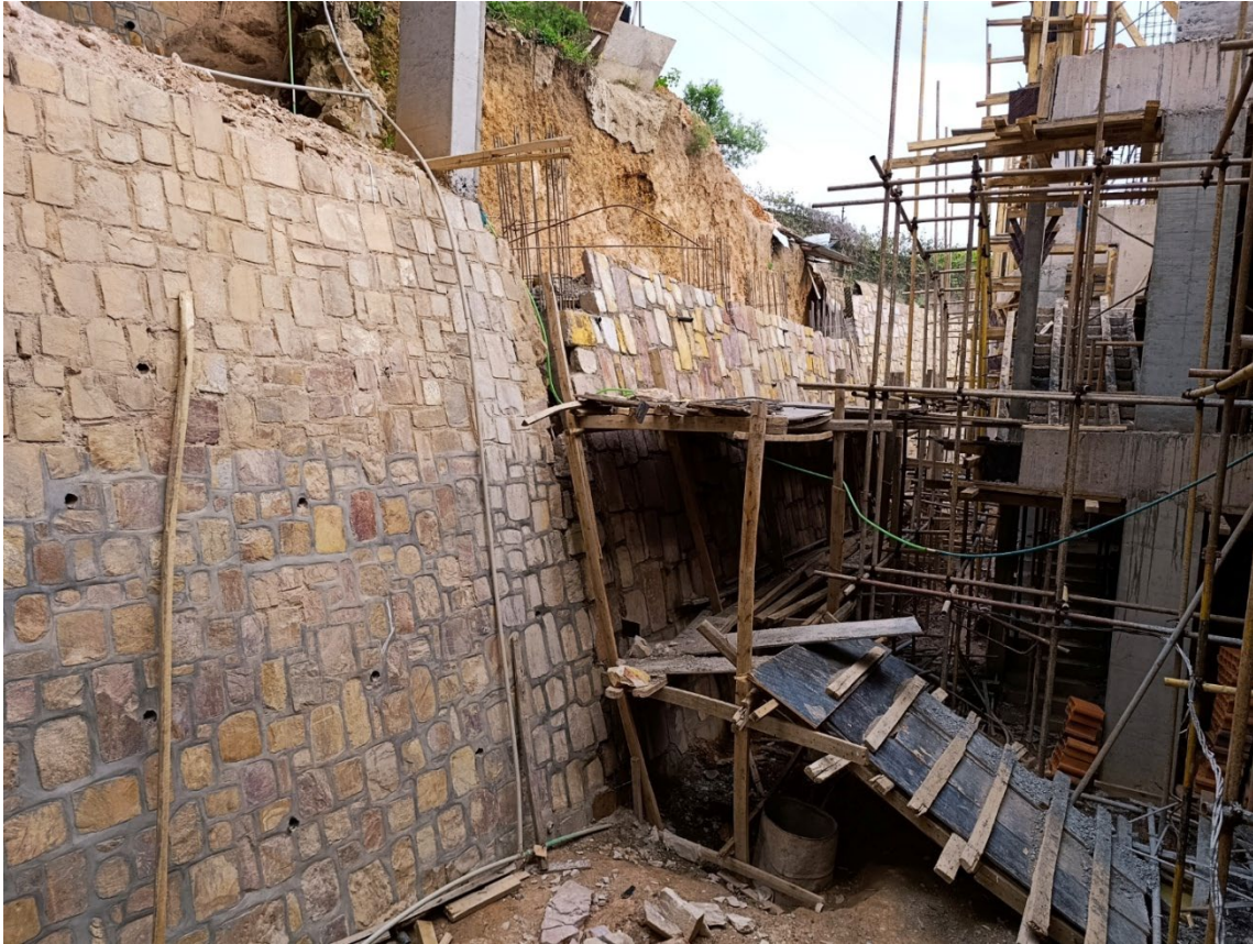
Phase 3 works showing: Masonry walling of retaining wall
