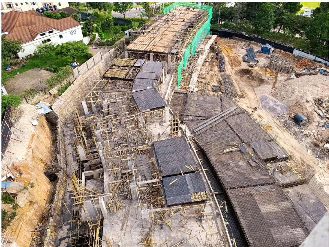
Phase 3/4 works showing: Formwork & steel reinforcement for slab on Lv. 4
