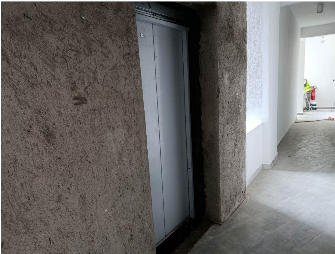
Phase 2 works showing: Installed lift doors in one of the lift lobbies
