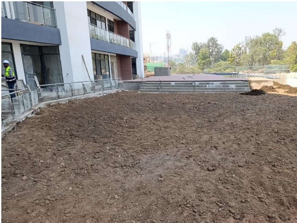
Phase 2 works showing: Soil filled on pool deck garden
