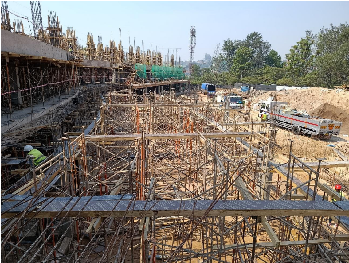
Phase 3 works showing: Formwork for pool deck slab
