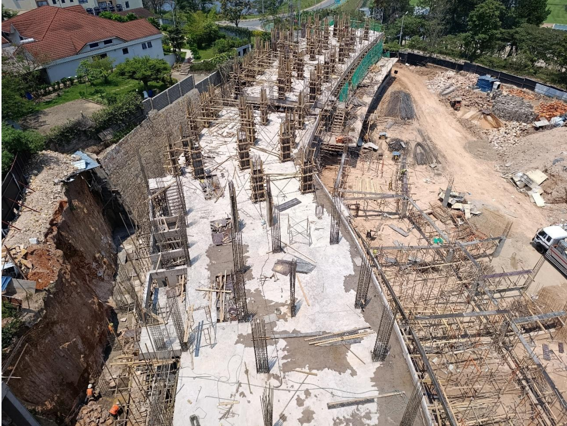
Phase 3/4 works showing: Formwork & steel reinforcement for columns on Lv. 3
