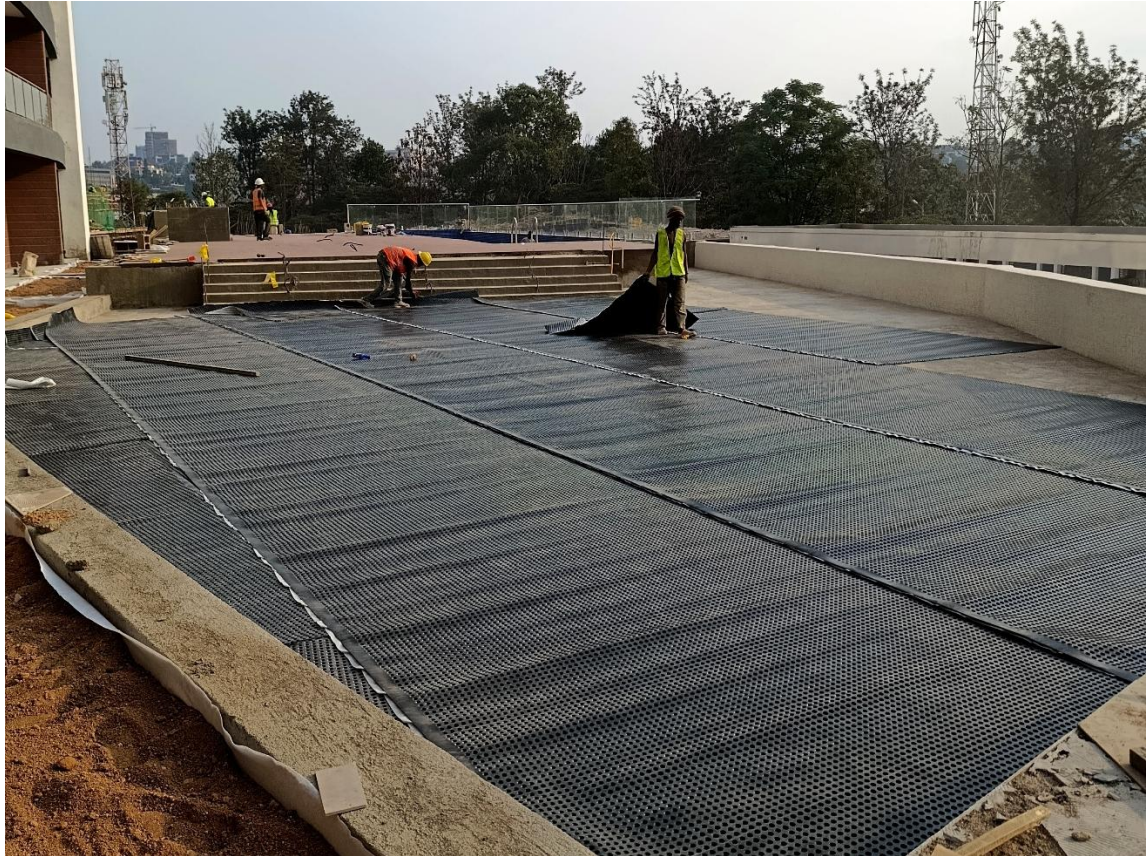
Phase 2 works showing: Waterproofing membrane fitted on pool deck garden
