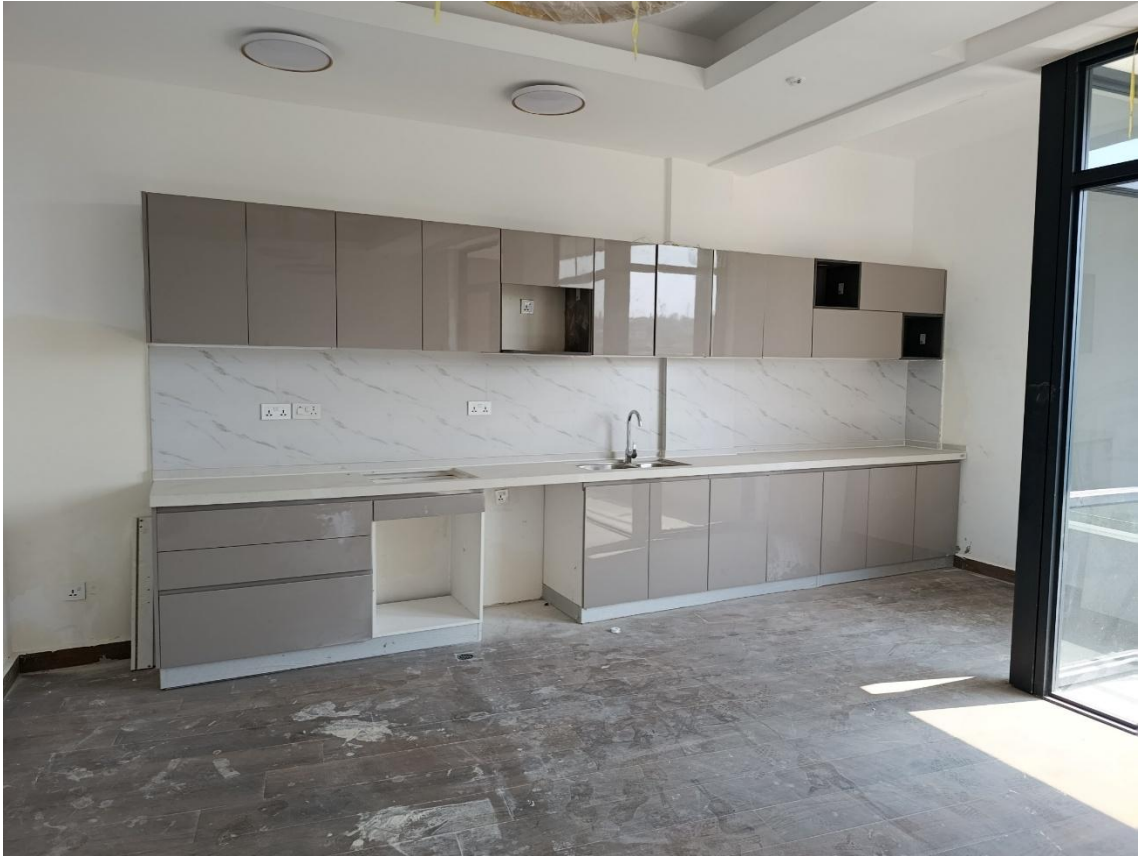
Phase 2 works showing: Kitchen walls tiled and socket installed in one of the units
