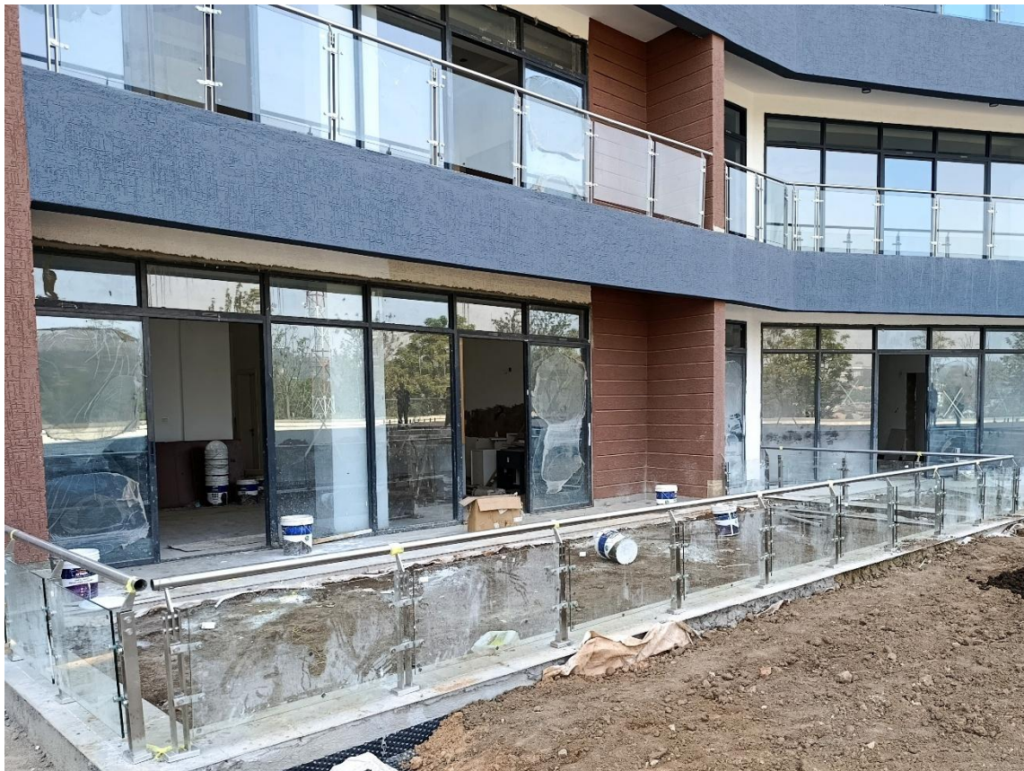
Phase 2 works showing: Balustrading fixed in one of the units on pool deck level
