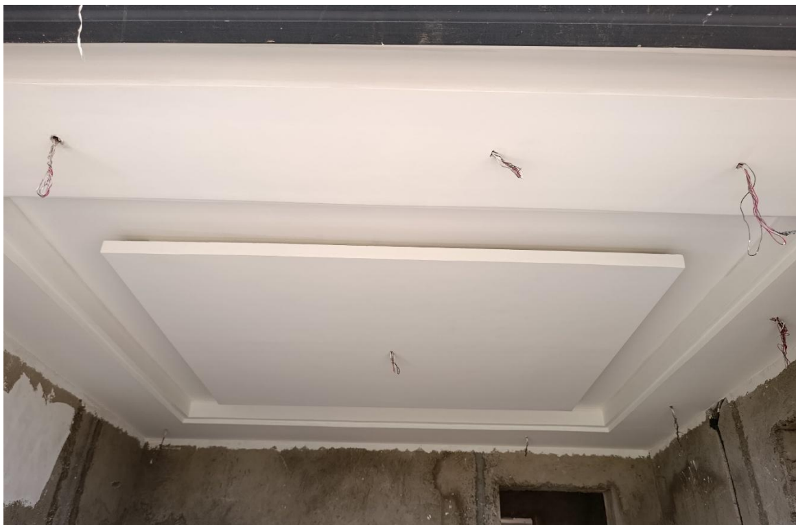
Phase 2 works showing: Gypsum ceiling one of the rooms at the penthouse
