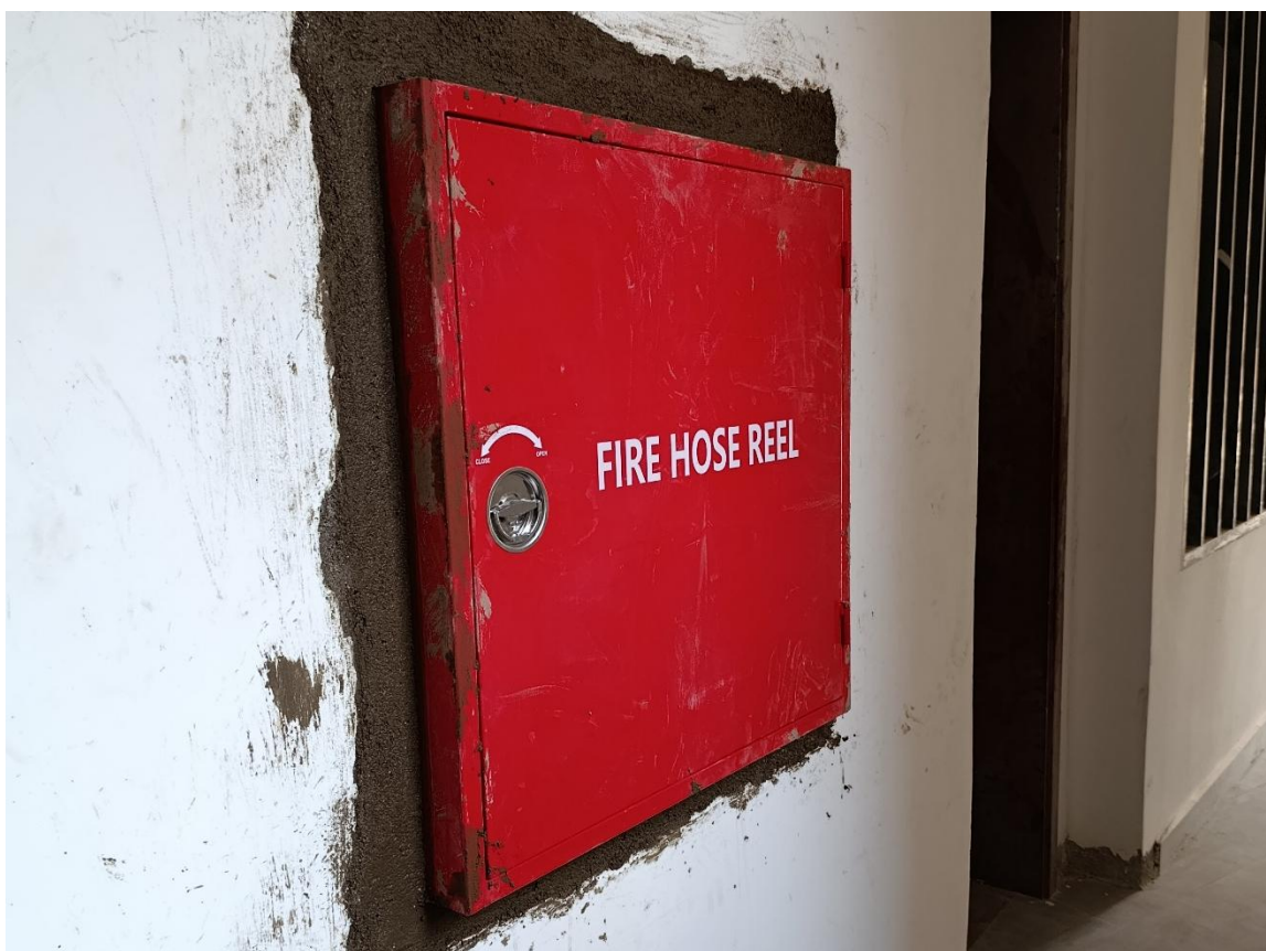
Phase 2 works showing: Fire hose-reel fitted in one of the corridors
