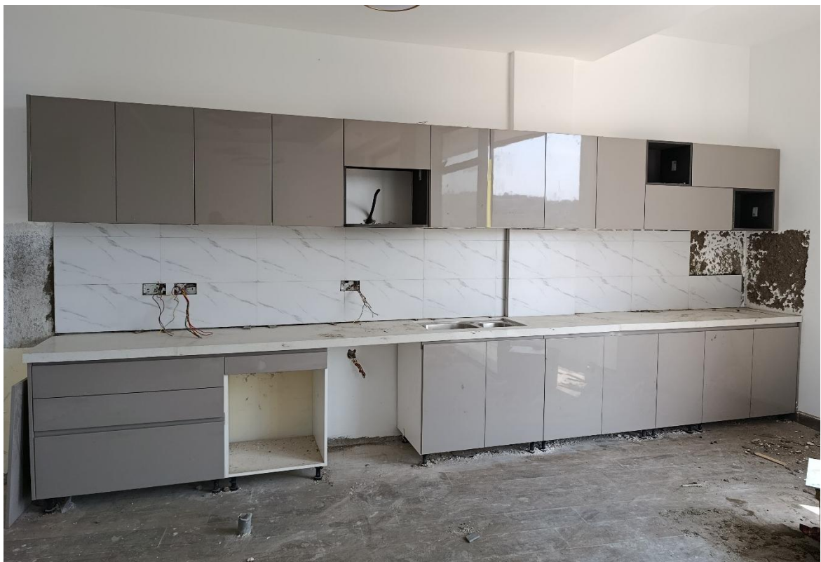
Phase 2 works showing: Kitchen cabinets & backsplash tiling in one of the units
