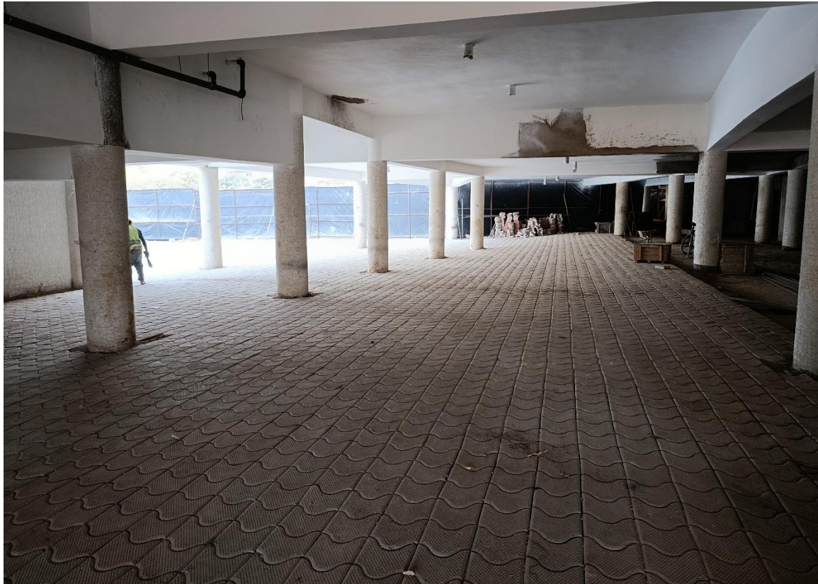
Phase 2 works showing: Parking area paving works
