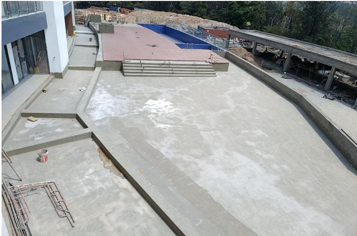
Phase 2 works showing: Waterproofing for garden & tiling on the swimming pool deck
