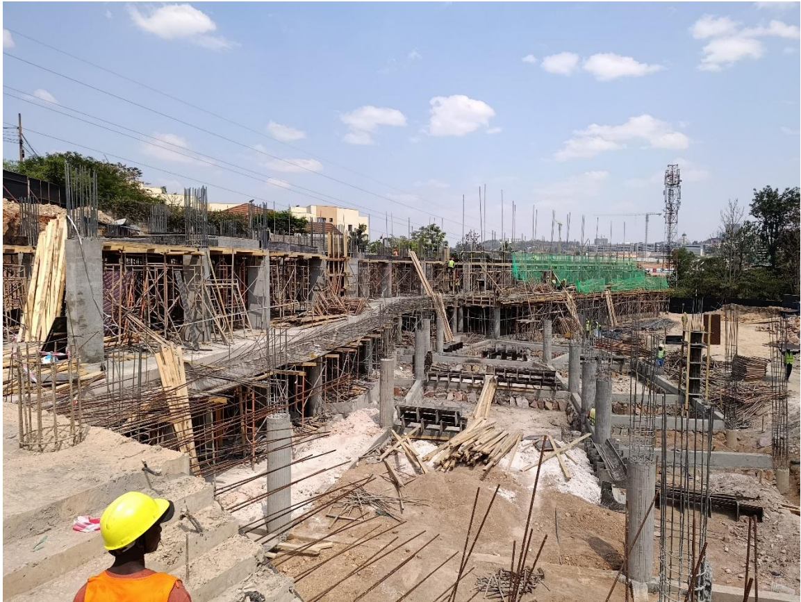
Phase 3/4 works showing: Formwork for second floor slab
