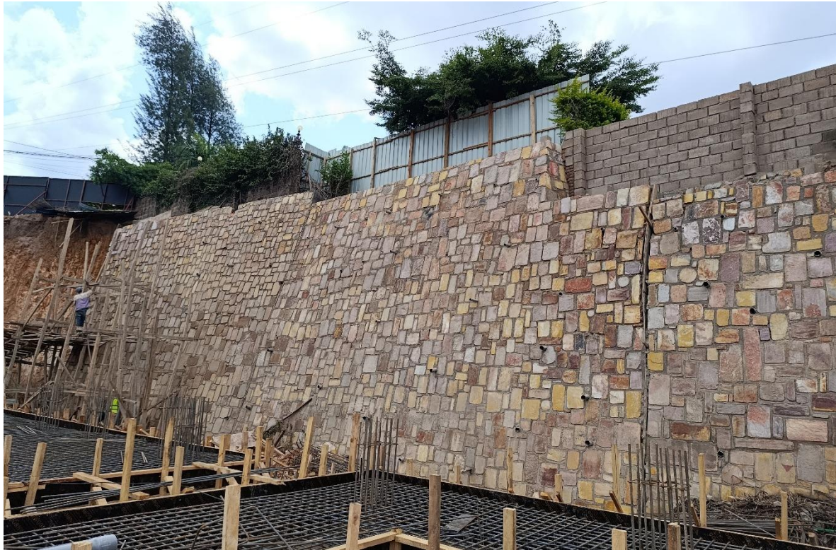
Phase 3 & 4 works showing: Stone masonry retaining wall
