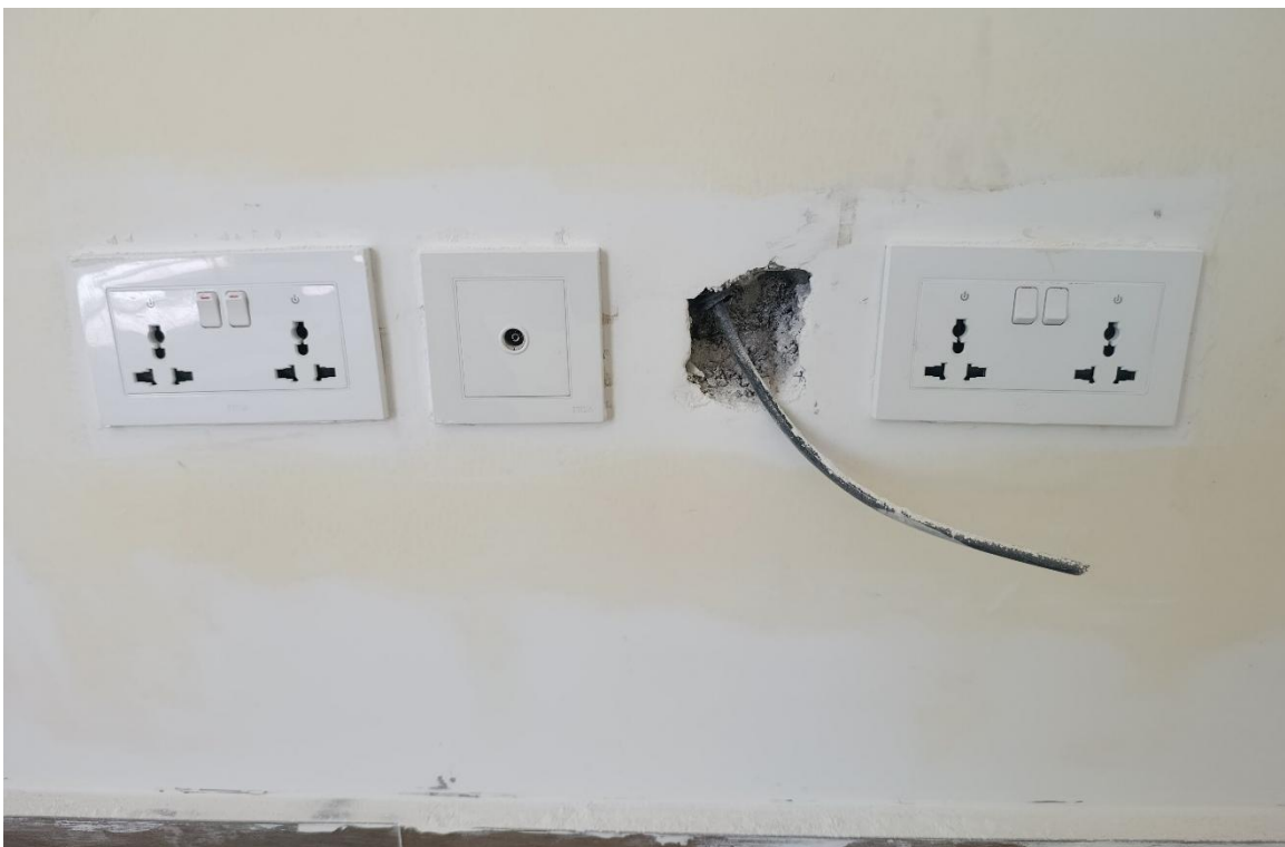
Phase 2 works showing: Socket outlets in one of the units
