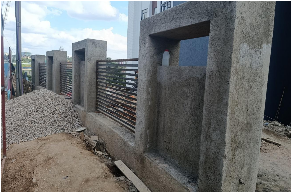
Phase 2 works showing: Masonry walling at the drop-off slab
