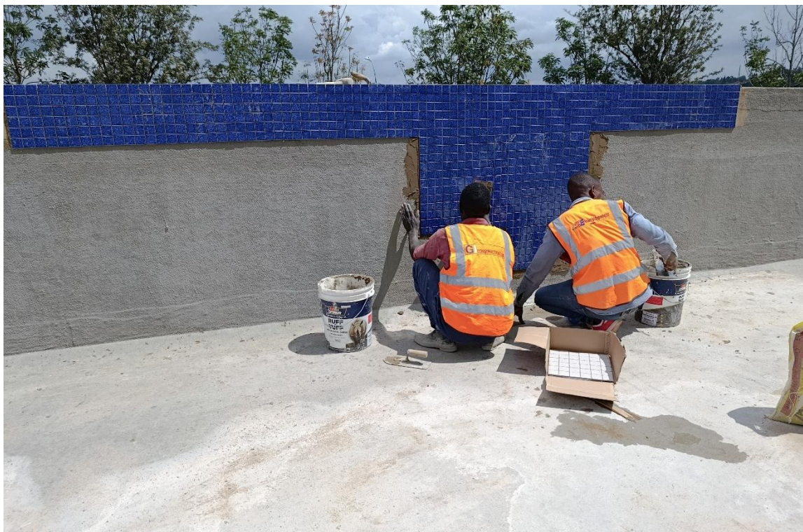
Phase 2 works showing: Tiling in swimming pool
