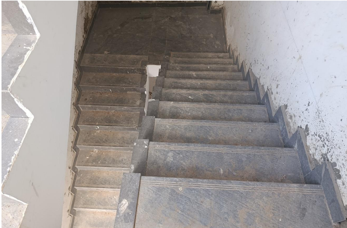
Phase 2 works showing: Tiling on staircase
