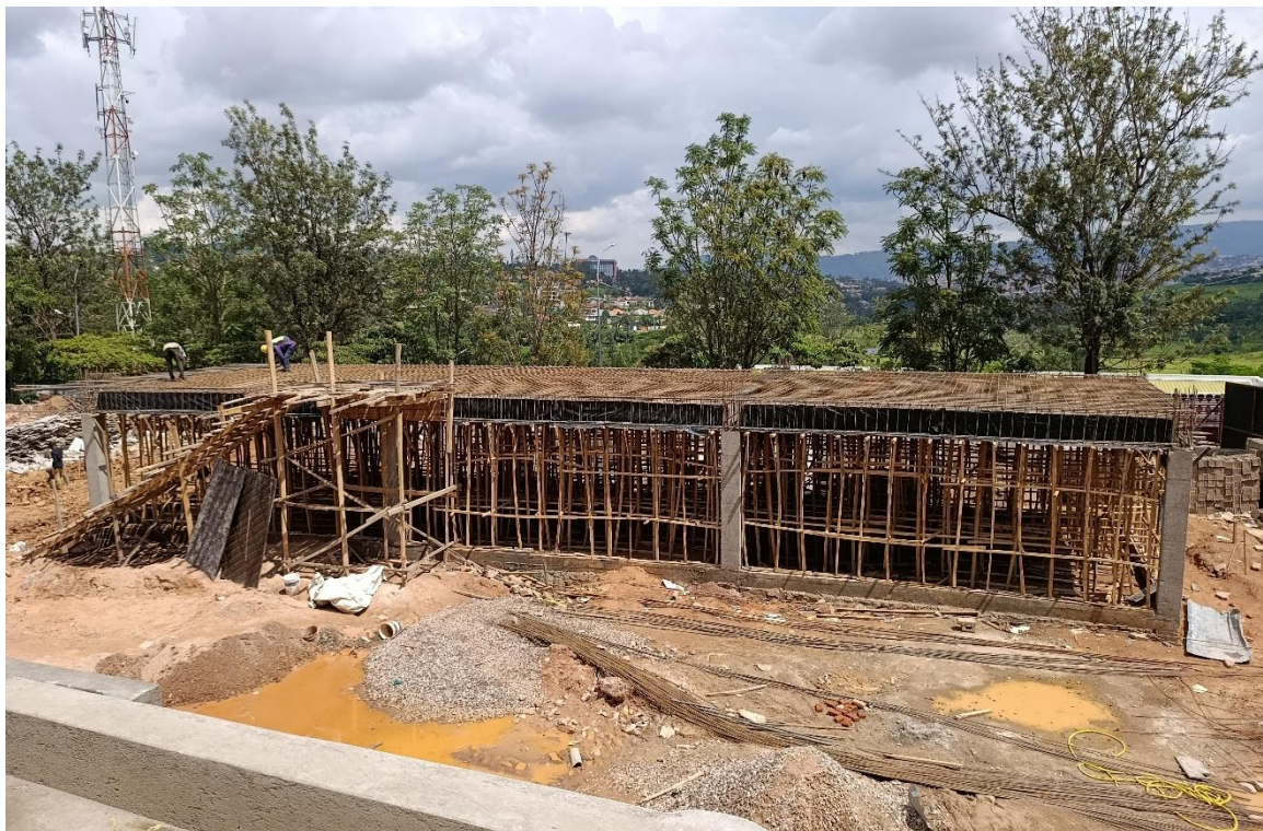
Phase 2 works showing: Steel reinforcement to cover slab of retail shops
