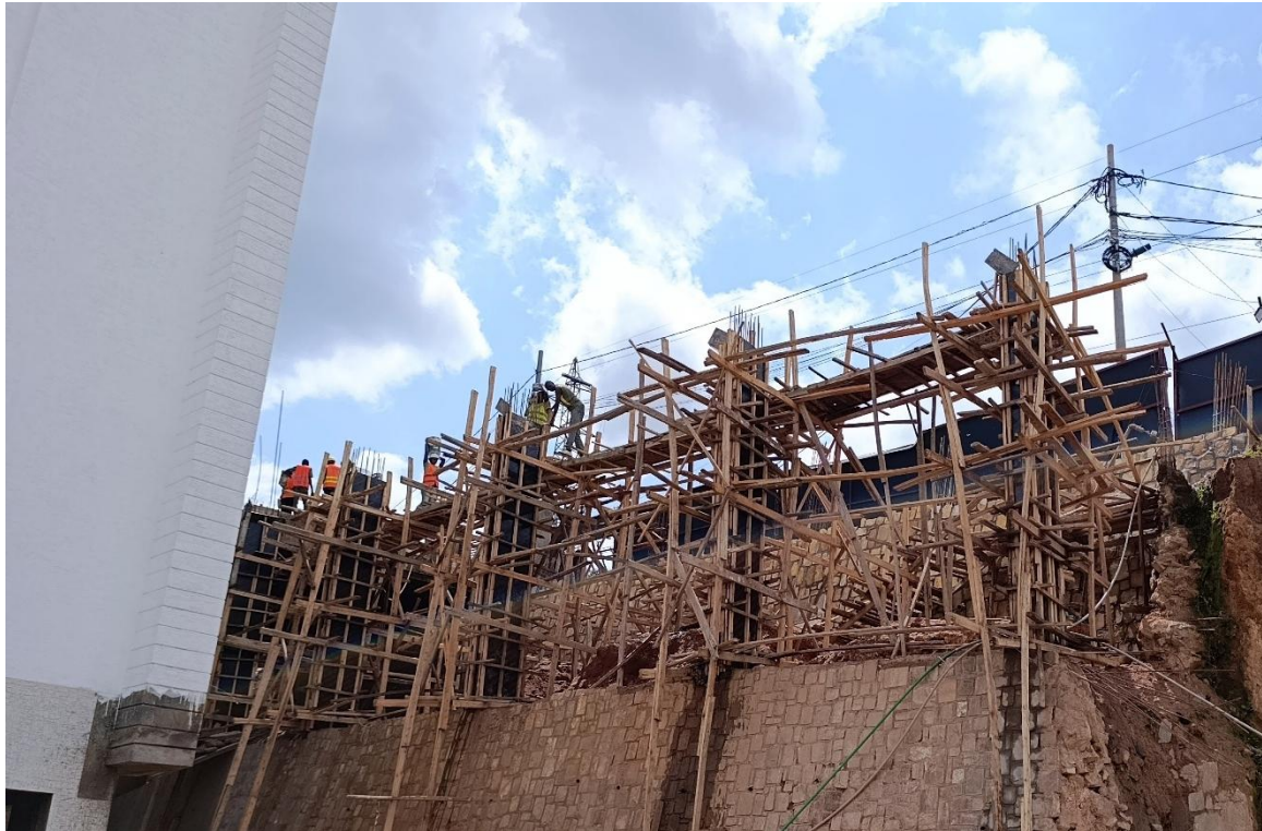
Phase 2 works showing: Formwork to columns for drop-off slab
