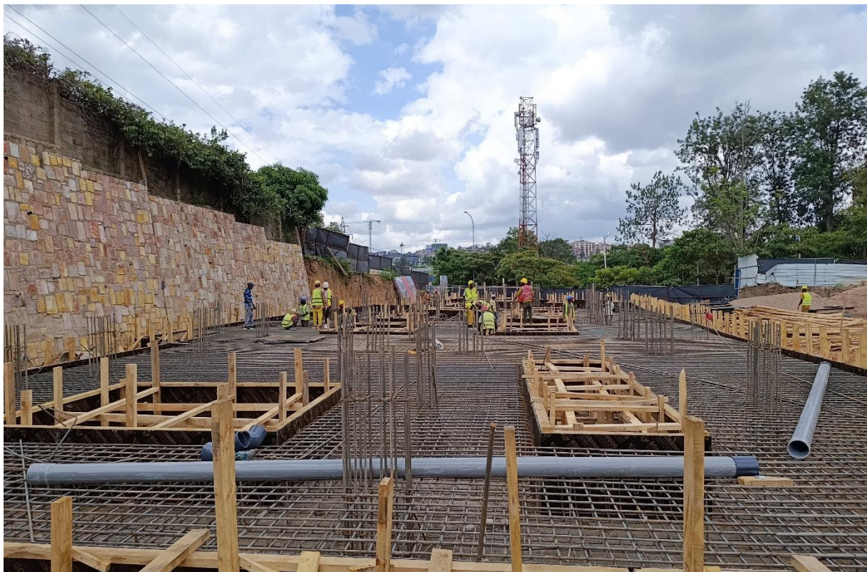
Phase 3 & 4 works showing: Steel reinforcement & Formwork for strip footing
