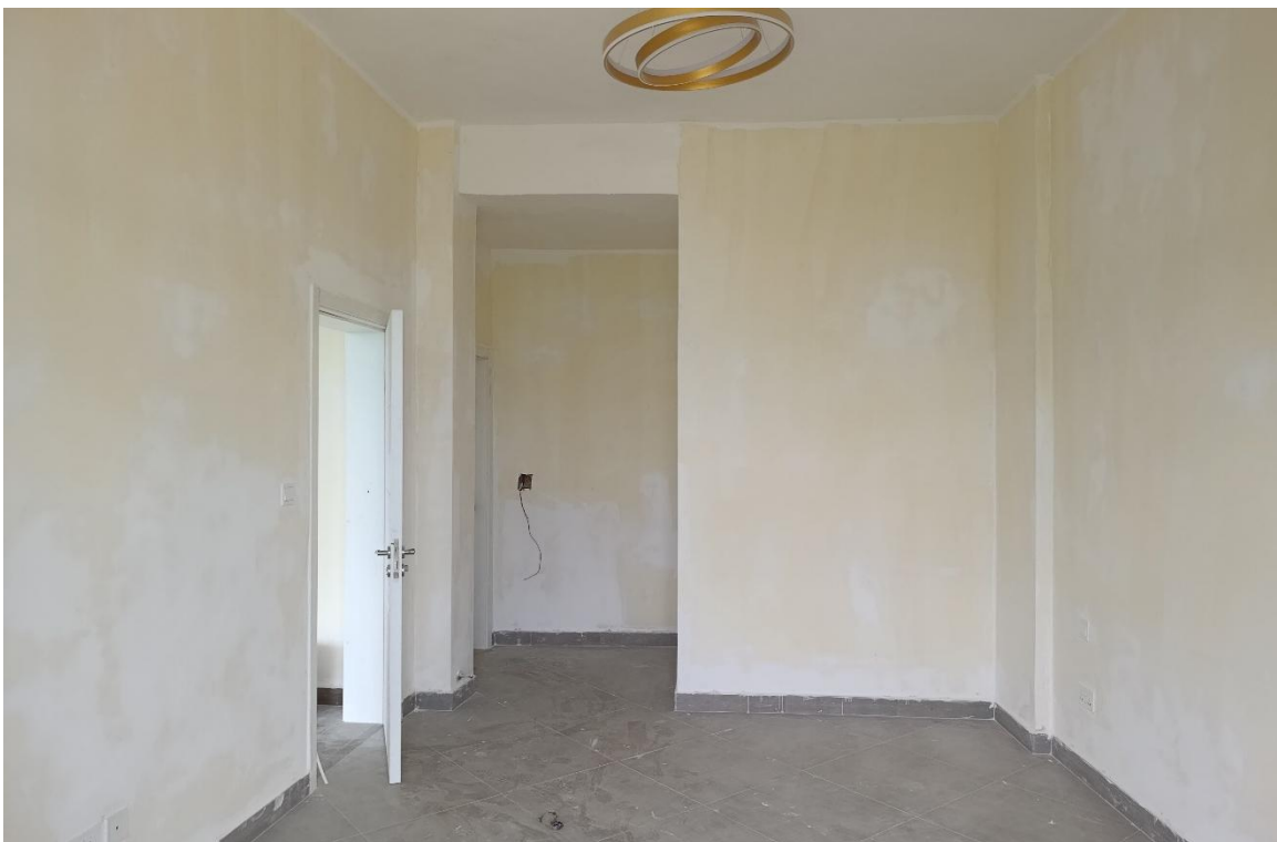
Phase 2 works showing: Skimming in one of the for one of the units
