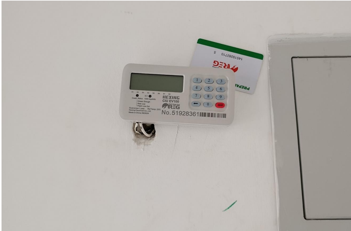
Phase 1 works showing: Cashpower meter installed in one of the units
