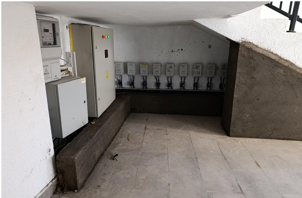
Phase 1 works showing: Distribution of main power to individual units
