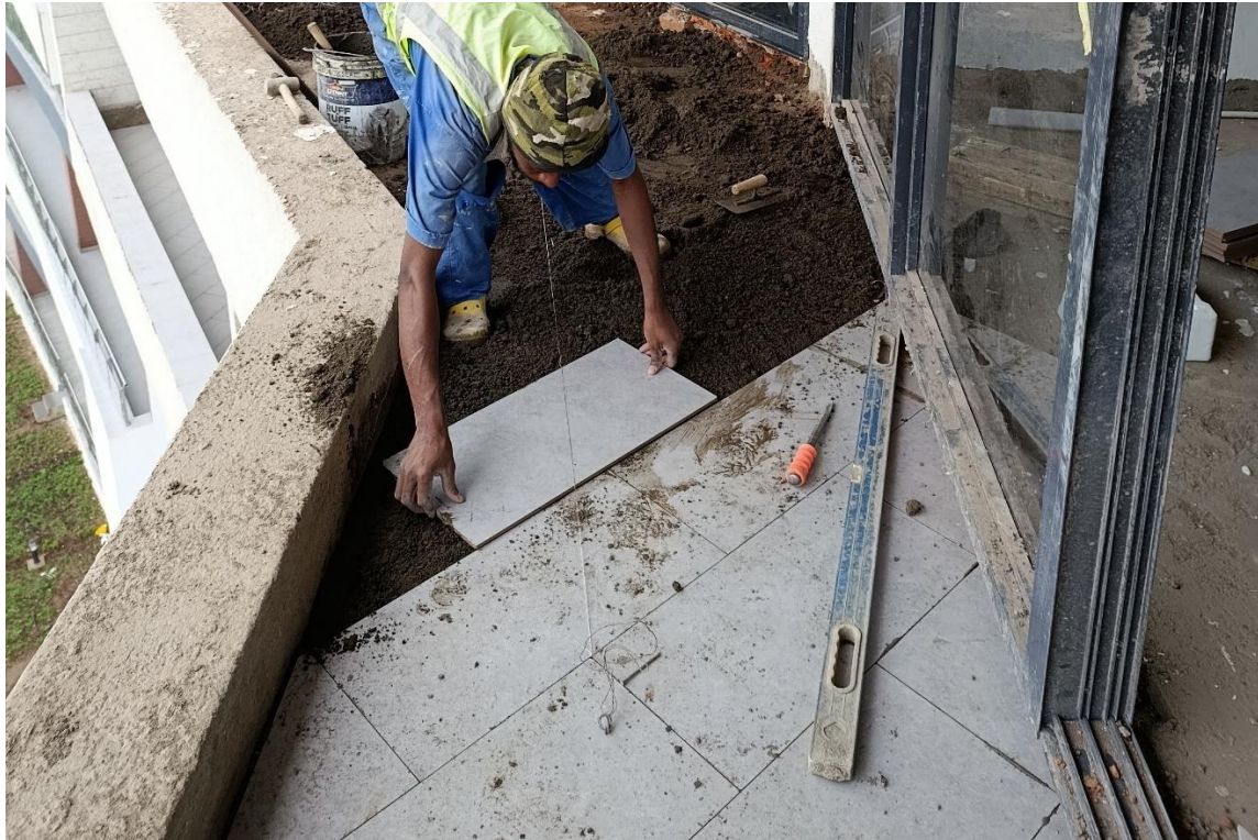
Phase 2 works showing: Floor tiling in the terrace one of the units
