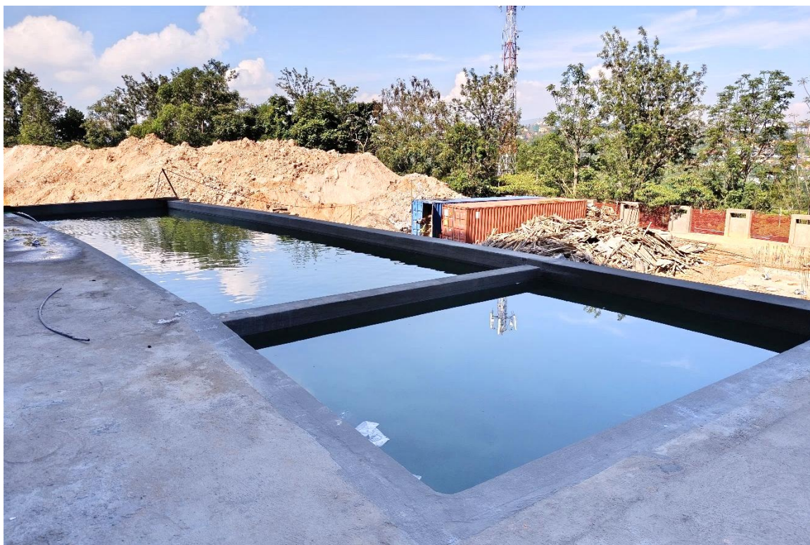
Phase 2 works showing: Testing of swimming pool for leakages before tilework
