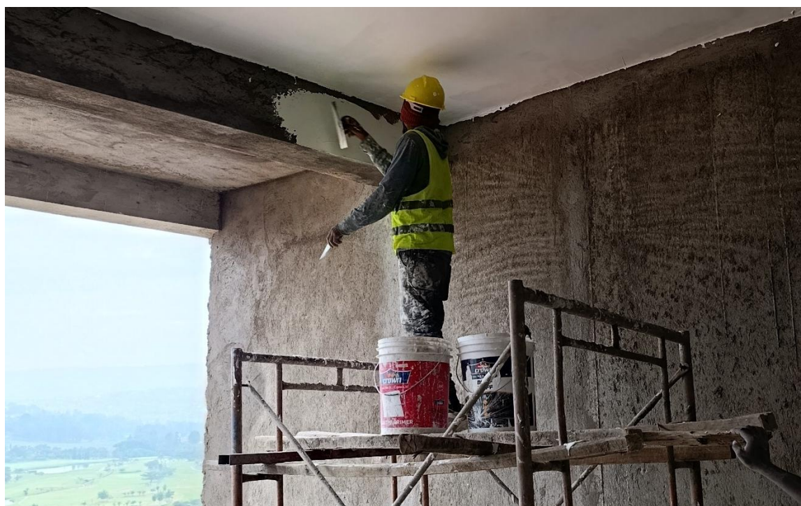
Phase 2 works showing: Internal wall skimming in one of the units
