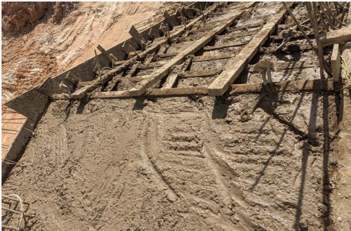
Phase 2 works showing: Cast concrete for staircase to pool deck
