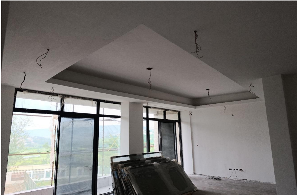
Phase 2 works showing: Skimmed gypsum ceiling with lighting wiring
