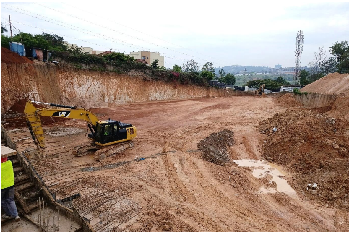
Phase 3/4 works showing: Excavated pit levelled and ready for setting-out
