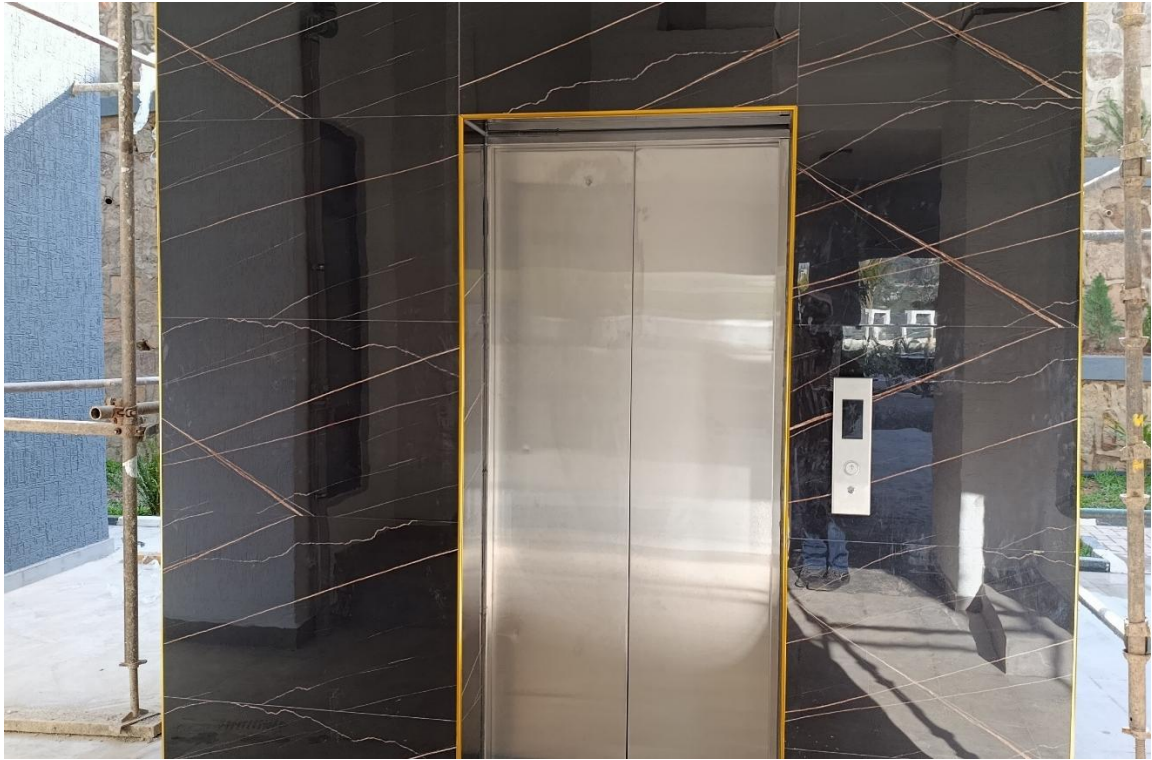
Phase 1 works showing: Granite finish and call-panel at lift lobby
