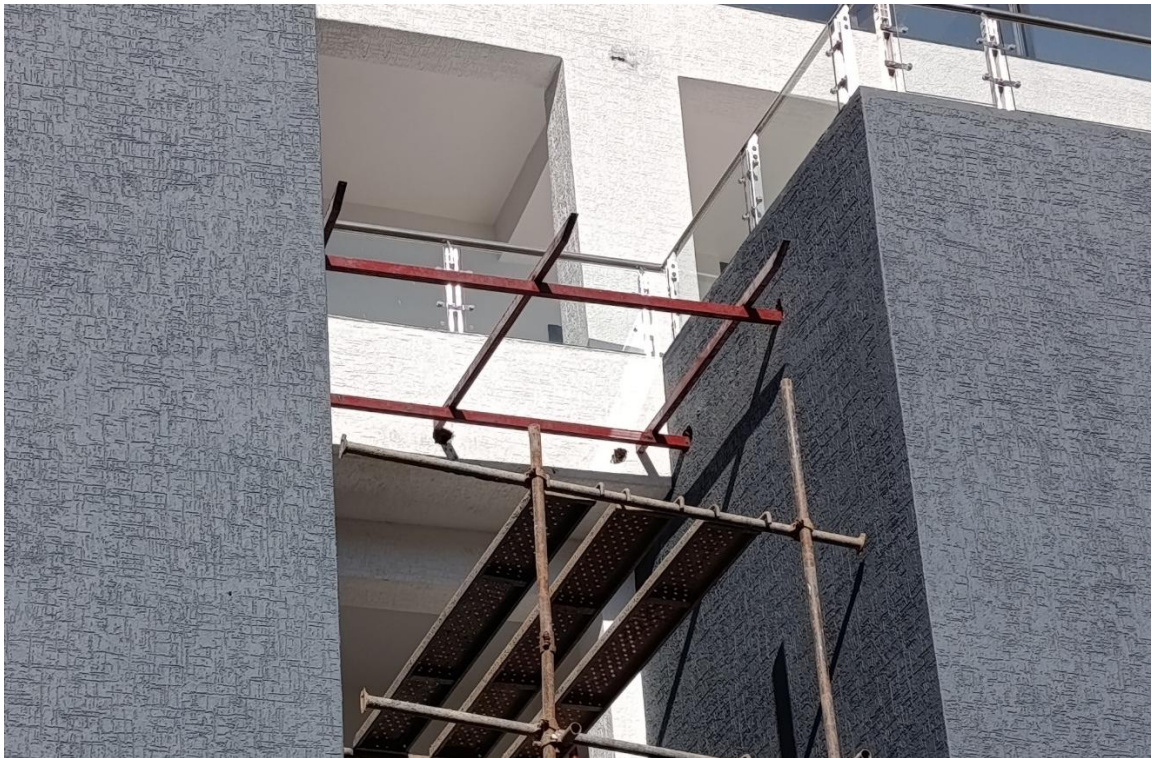
Phase 1 works showing: Framing for canopy to shield balconies from rain
