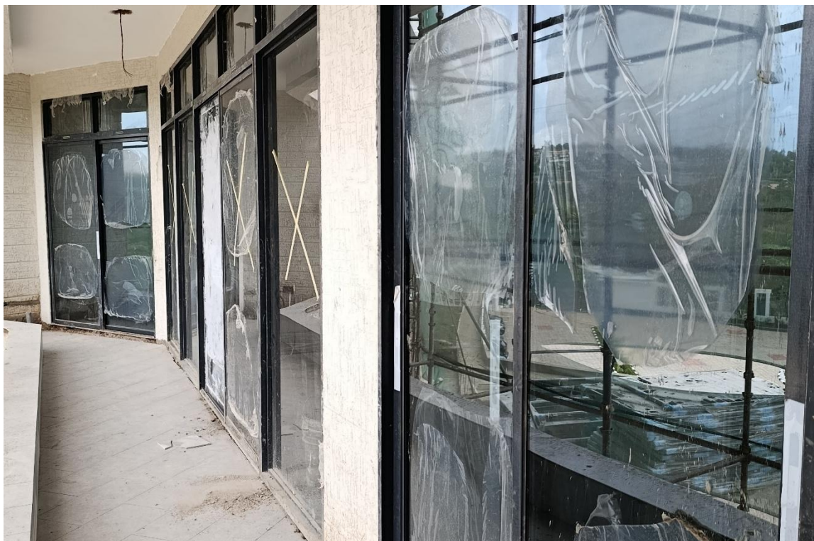
Phase 2 works showing: Curtain wall glazing installed in one of the units
