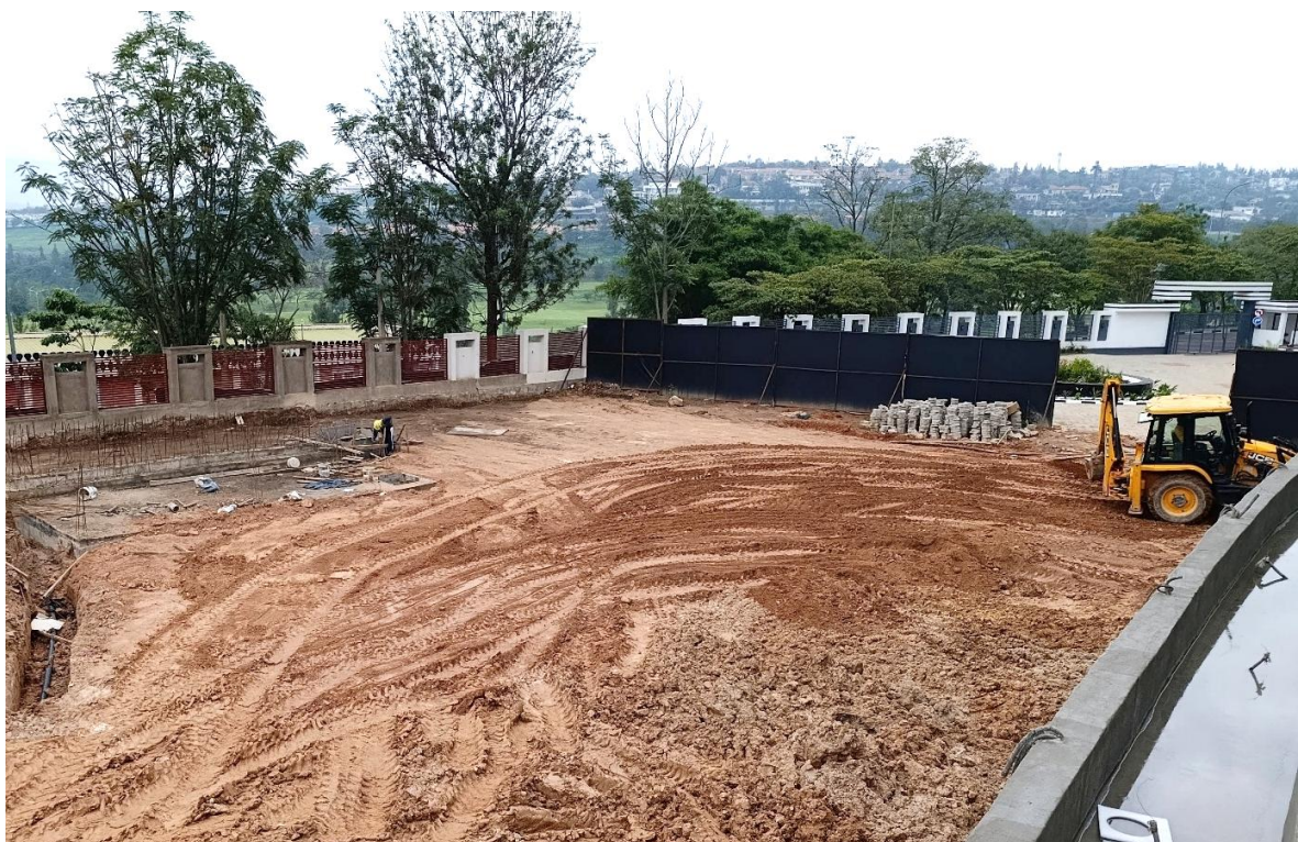
Phase 1/2 works showing: Backfill and compaction in preparation for paving
