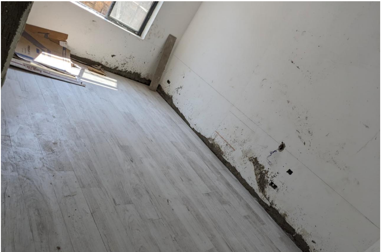
Phase 2 works showing: Floor tiling in one of the units
