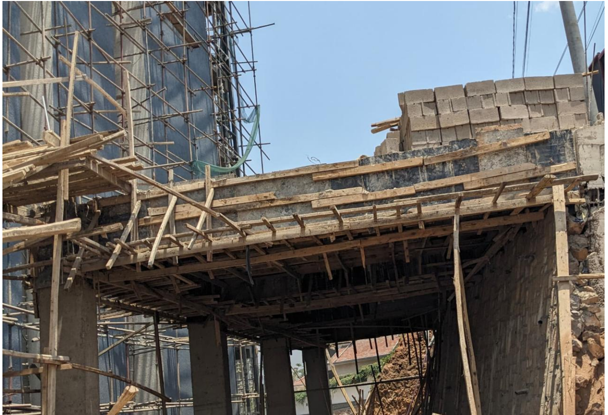
Phase 1 works showing: Part of cast drop-off slab
