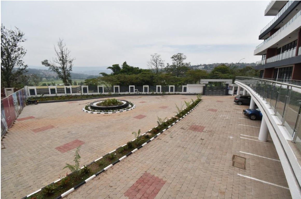
View of Phase 1 parking from phase 2 pool deck
