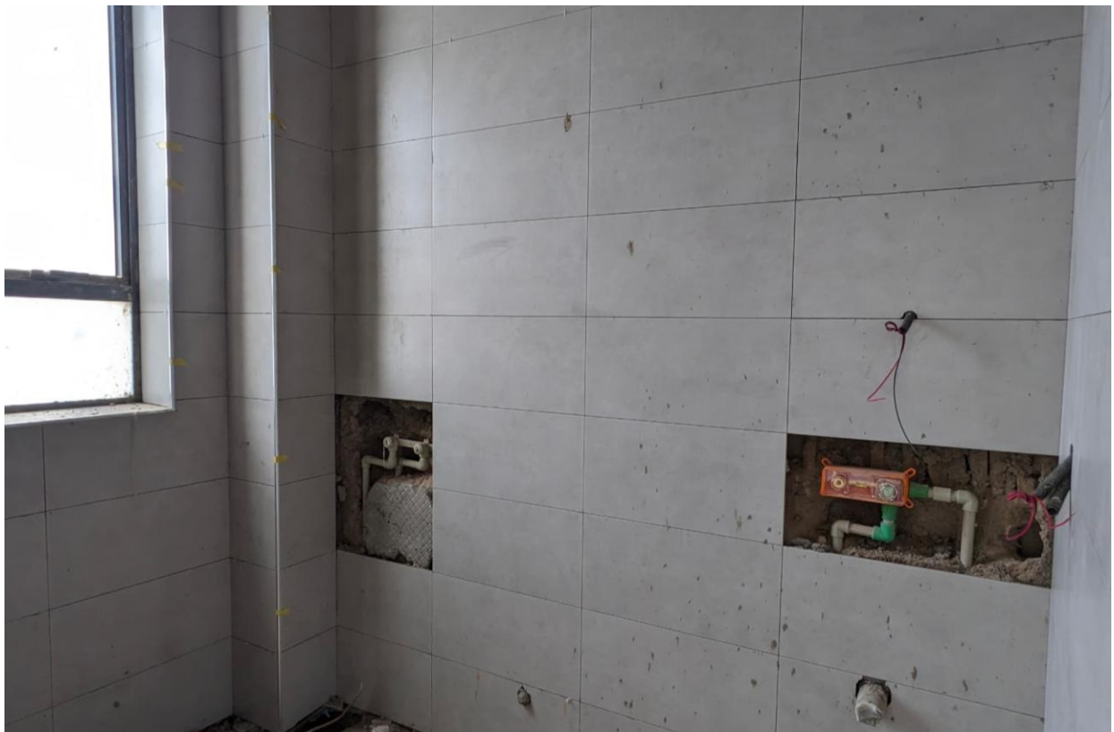
Phase 2 works showing: Wall tiling in one of the washrooms
