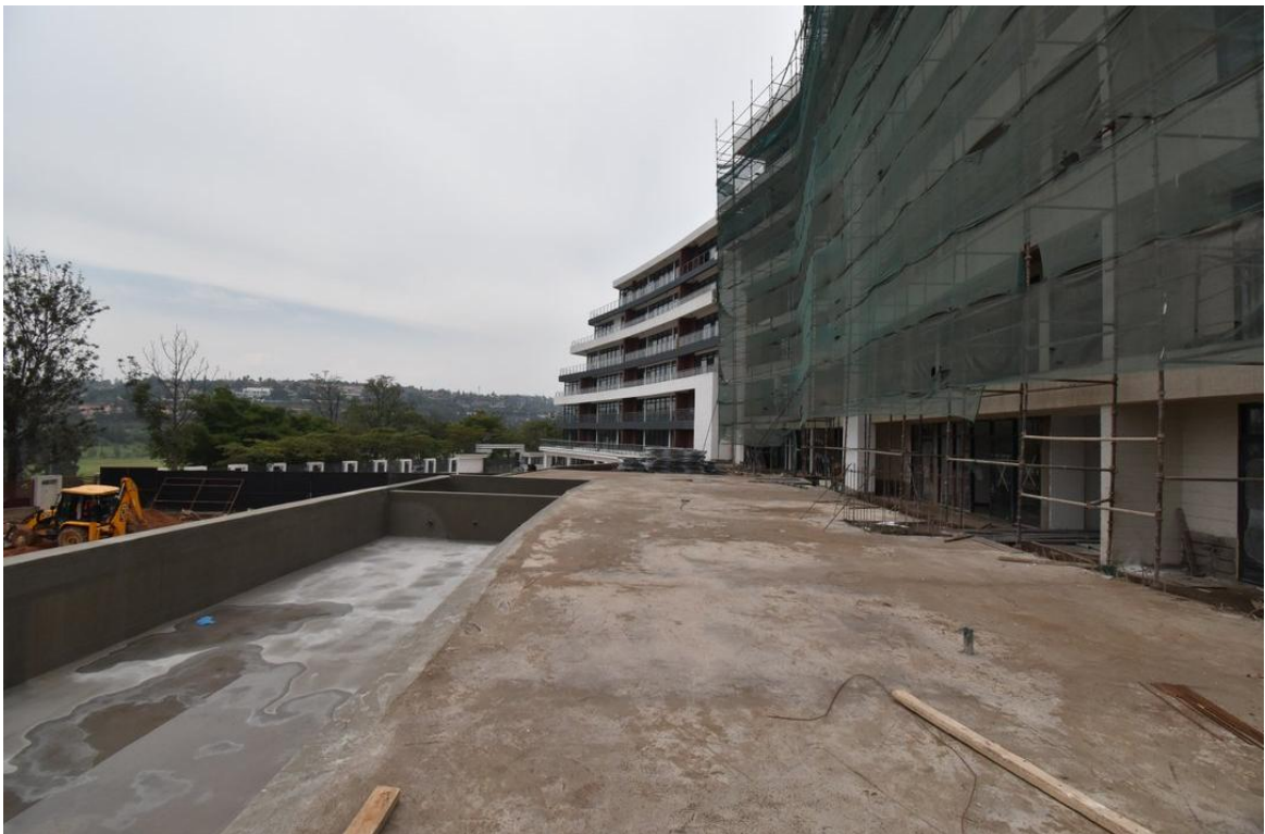
Phase 1 and 2 seen from the pool deck
