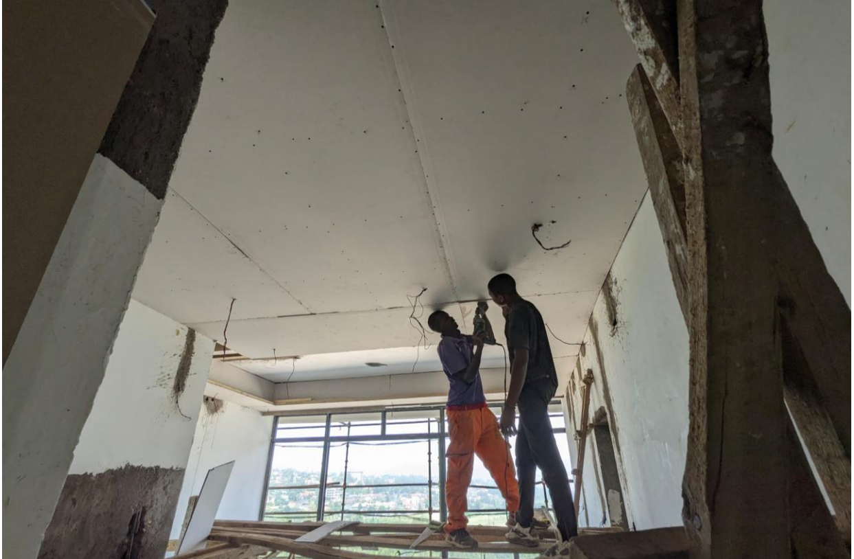
Phase 2 works showing: Gypsum ceiling installation in one of the units
