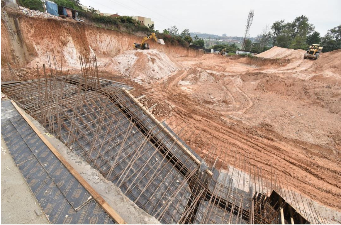
Staircase between Phase 2 and 3
