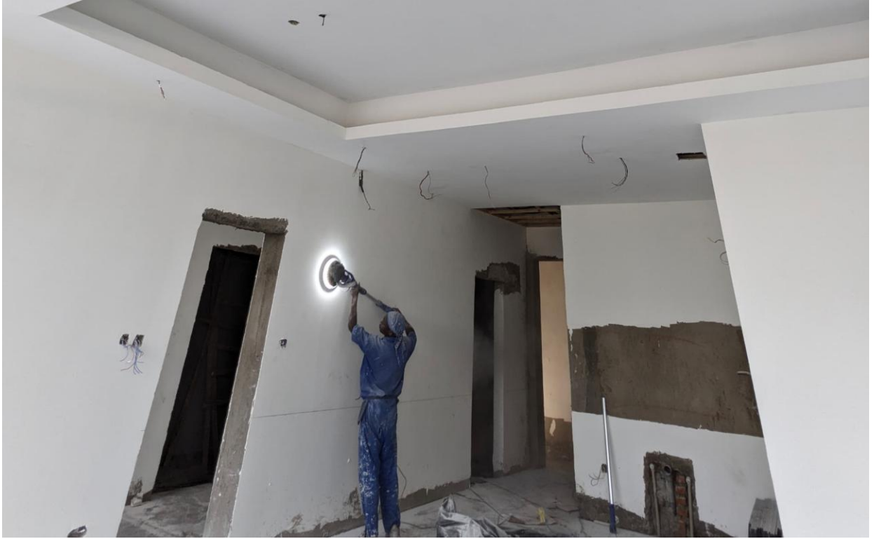
Phase 2 works showing: Internal wall skimming
