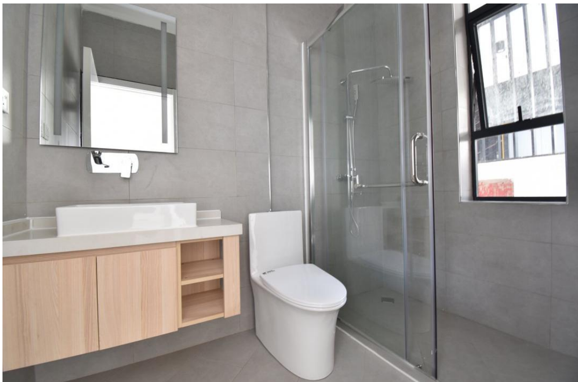
Finished bathroom, phase 1
