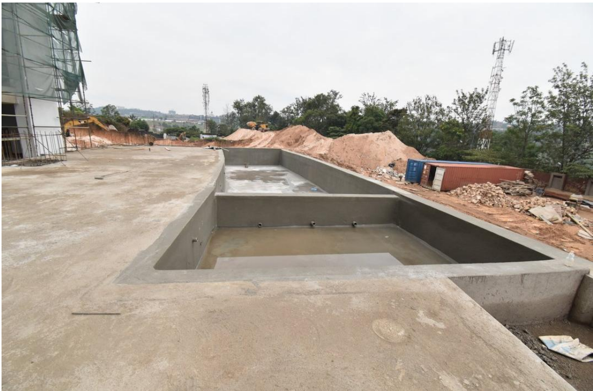
Phase 2 showing the pool, water proofing done
