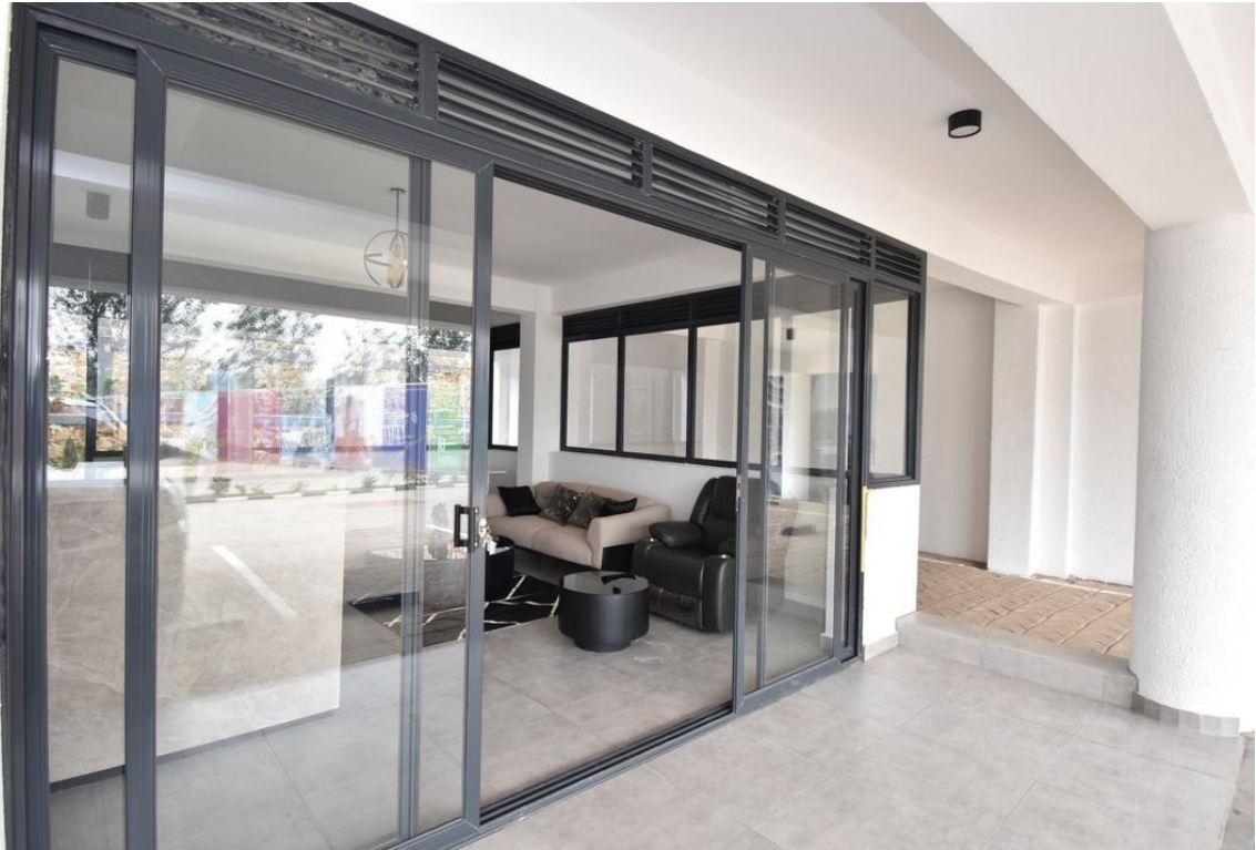
View of Phase 1 reception from outside
