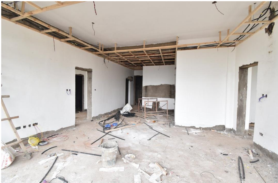
One of the units in Phase 2, with painting ongoing.
