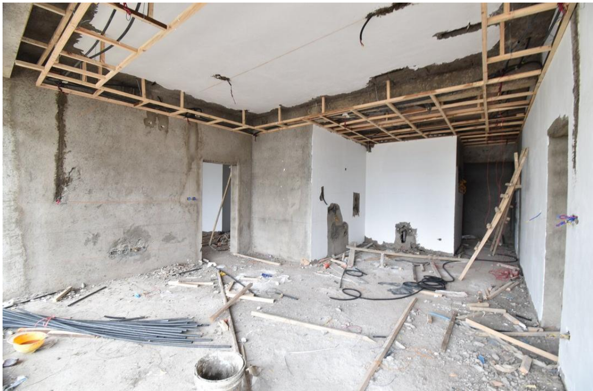
One of the Phase 2 units, showing plastering works done and painting
