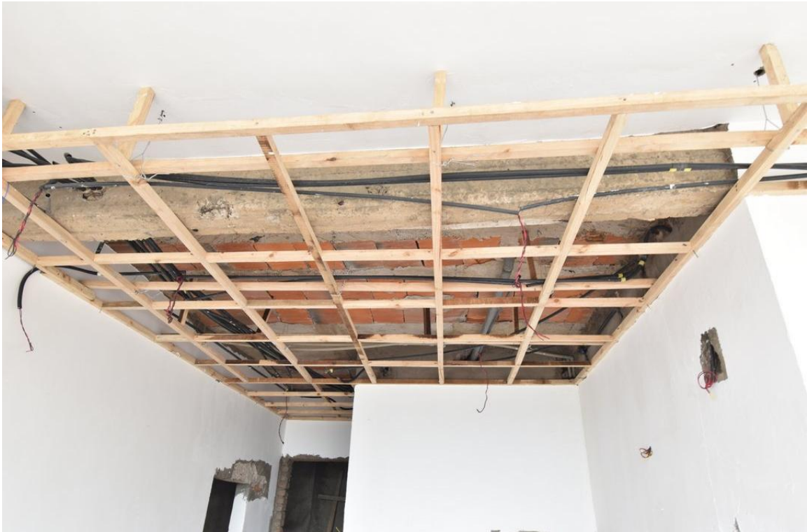
Phase 2 gypsum blundering ongoing.
