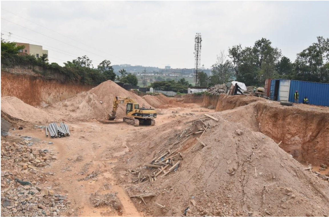
Phase 3 & 4 works showing: Mass excavation to reduce soil levels to Basement 3
