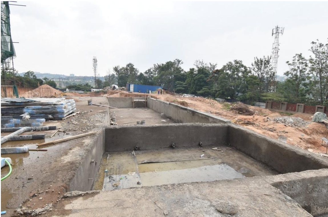
Phase 2 swimming pool, plaster works done
