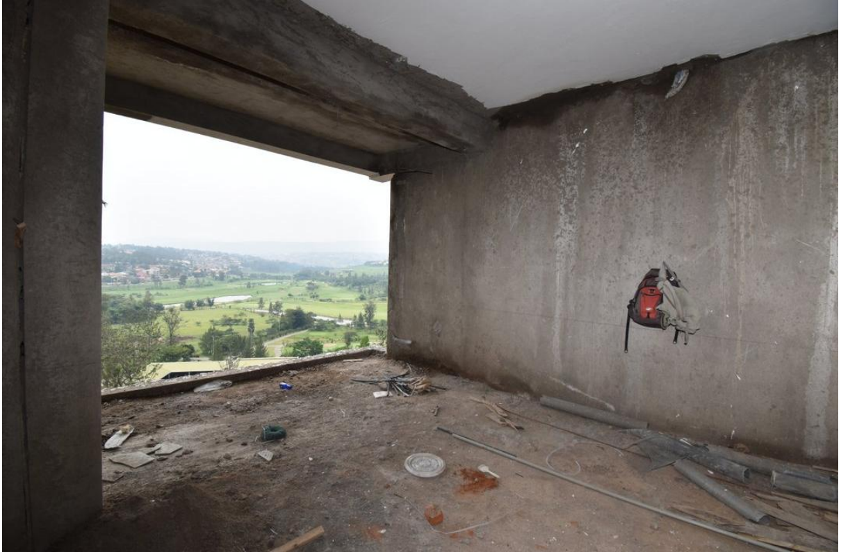
Works in one of the units in Phase 2
