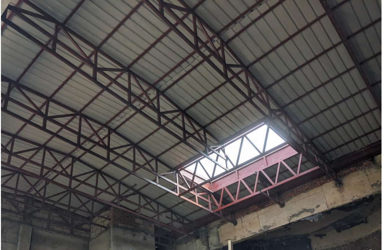
Phase 2 works showing: Roof truss installed in Lv. 2 of penthouse
