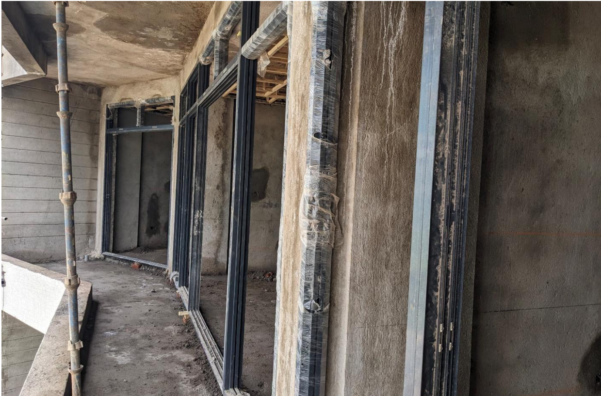
Phase 2 works showing: Curtain wall installed in one of the units
