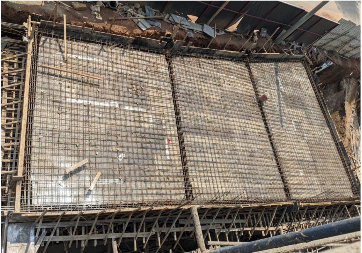
Phase 2 works showing: Steel reinforcement for drop-off slab
