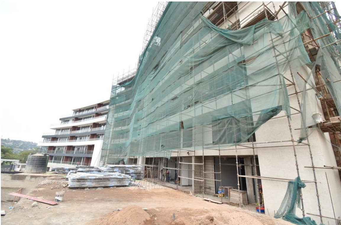
Phase 1 and 2, seen from the pool deck
