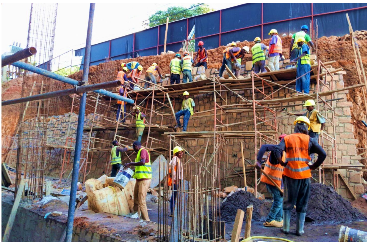
Phase 2 works showing: Masonry walling in Lv. 2 of retaining wall
