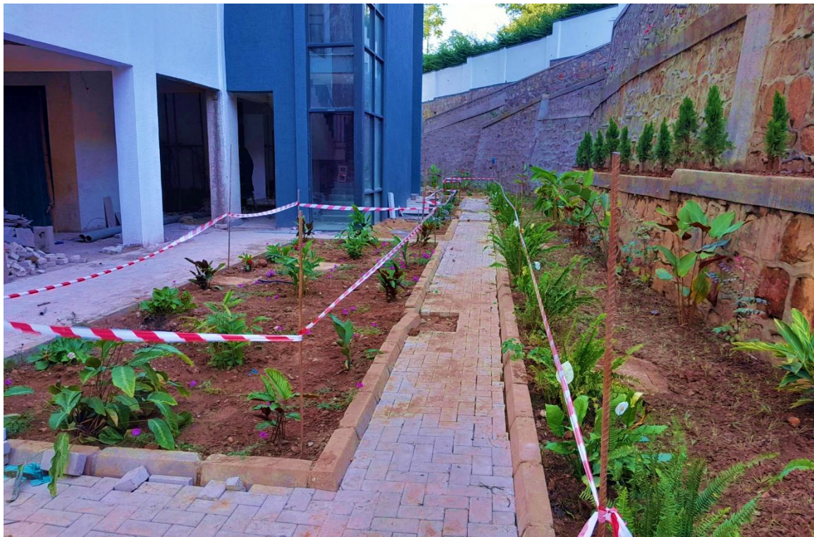
Phase 1 works showing: Landscaped backyard
