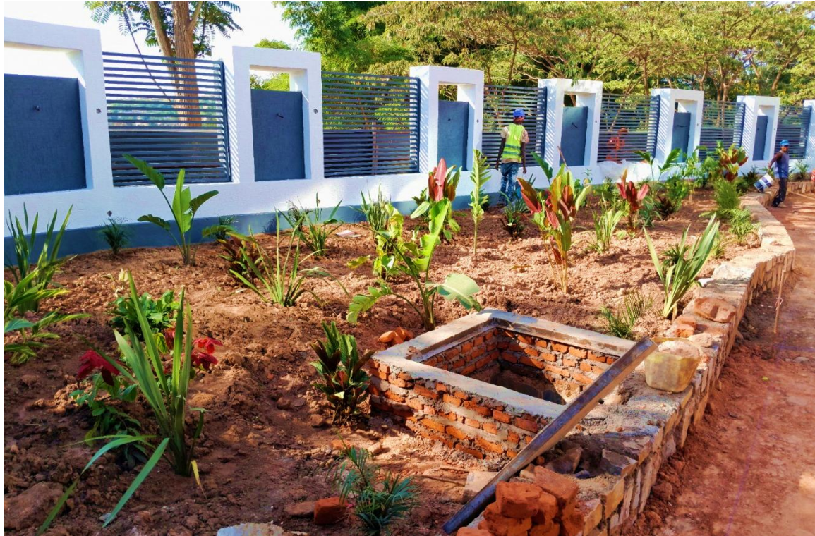
Phase 1 works showing: Planted greenery in the garden
