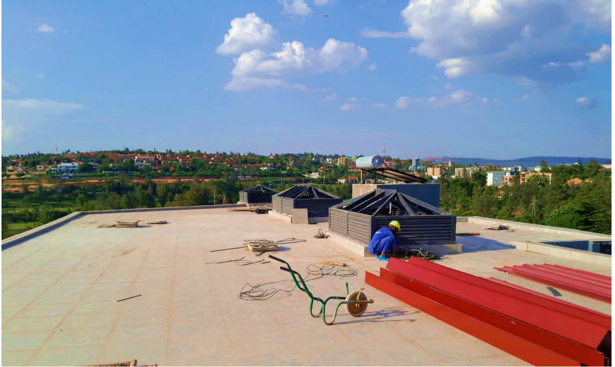
Phase 1 works showing: Vents installed at the roof terrace
