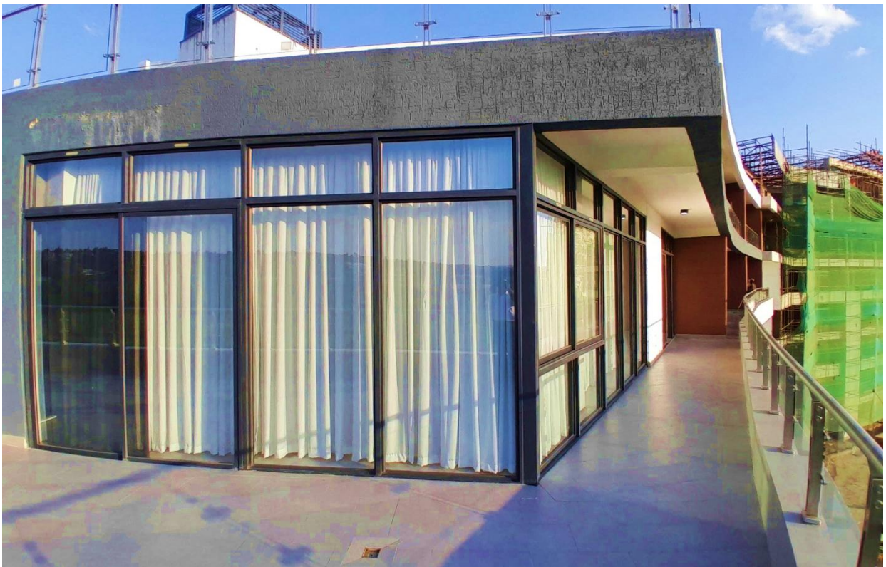
Phase 1 works showing: Finished balcony in one of the units
