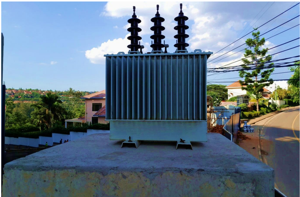
Phase 1 works showing: Installed transformer
