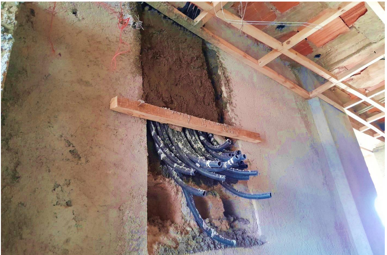
Phase 2 works showing: Internal electrical conduiting in one of the units
