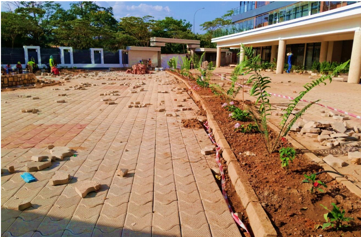
Phase 1 works showing: Laying of pavers in parking.
