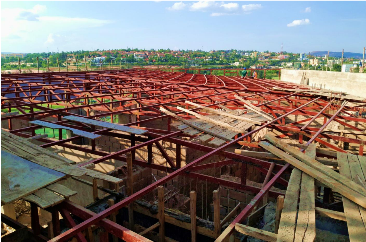
Phase 2 works showing: Roof truss installed in Lv. 1 of penthouse
