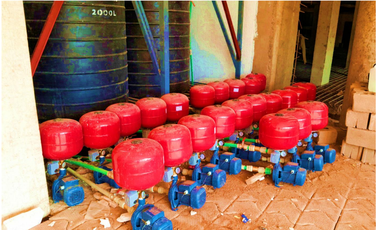
Phase 1 works showing: Installed water pumps
