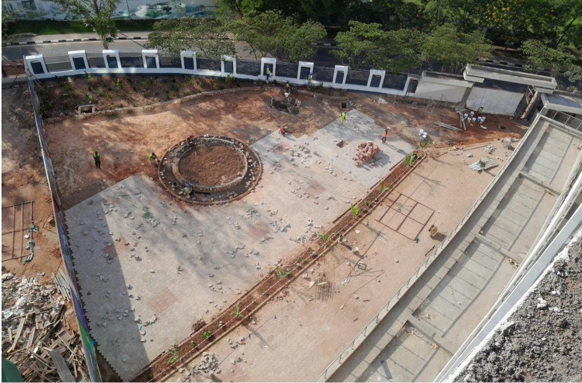
Phase 1 works showing: Bird's eye view of parking and garden
