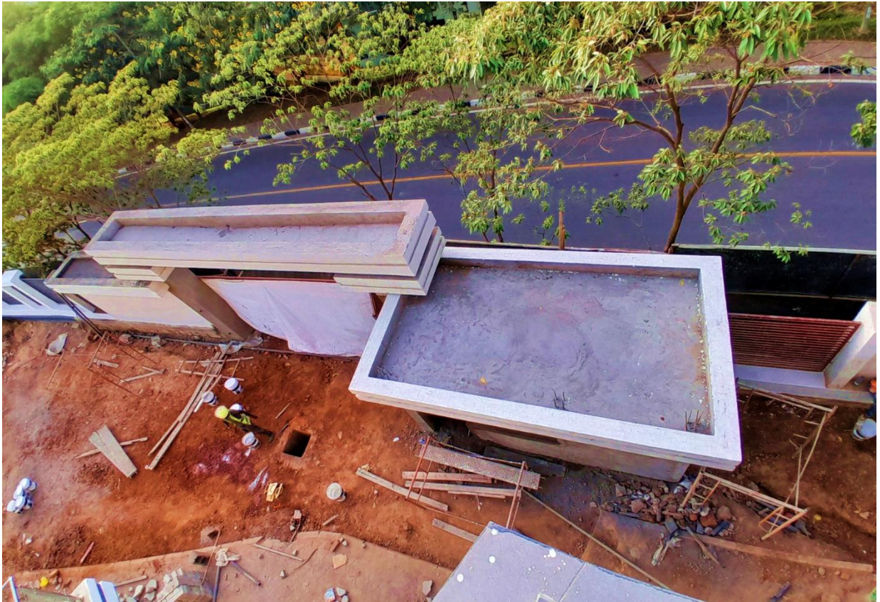
Phase 1 works showing: Gate & guard house
