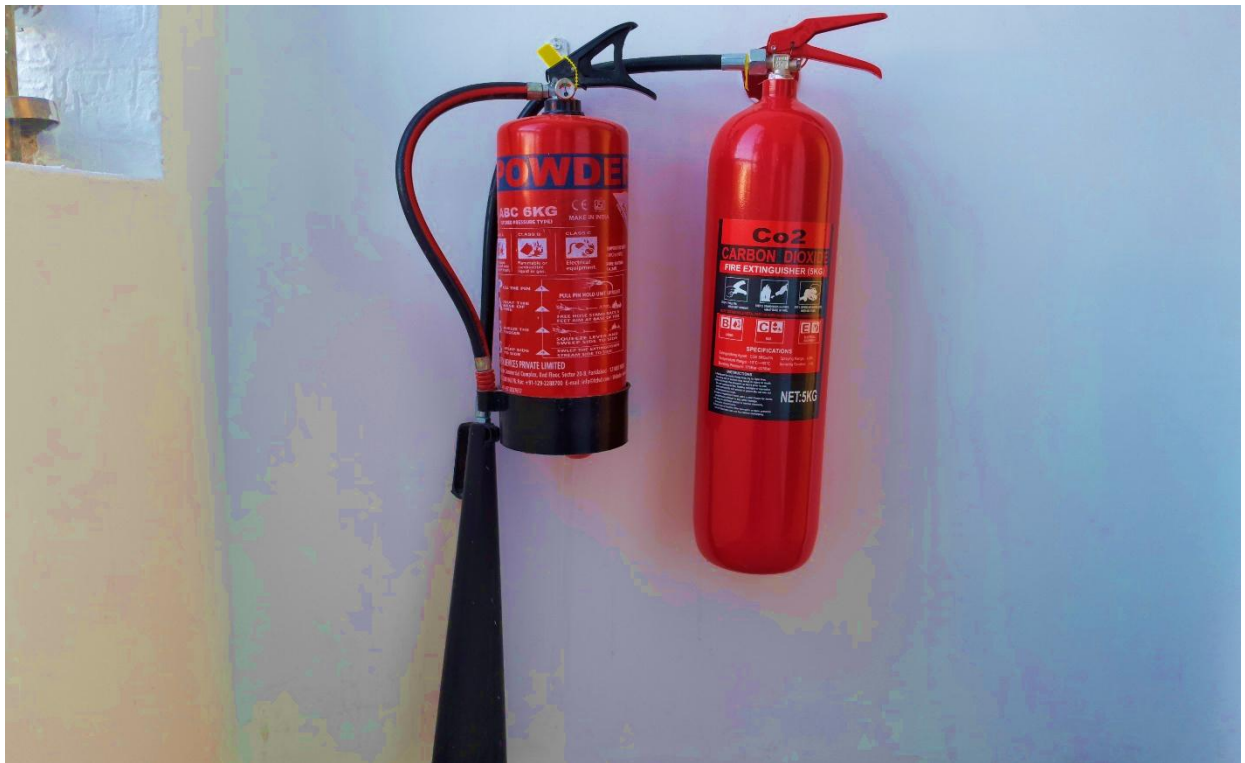
Phase 1 works showing: Fire extinguishers installed
