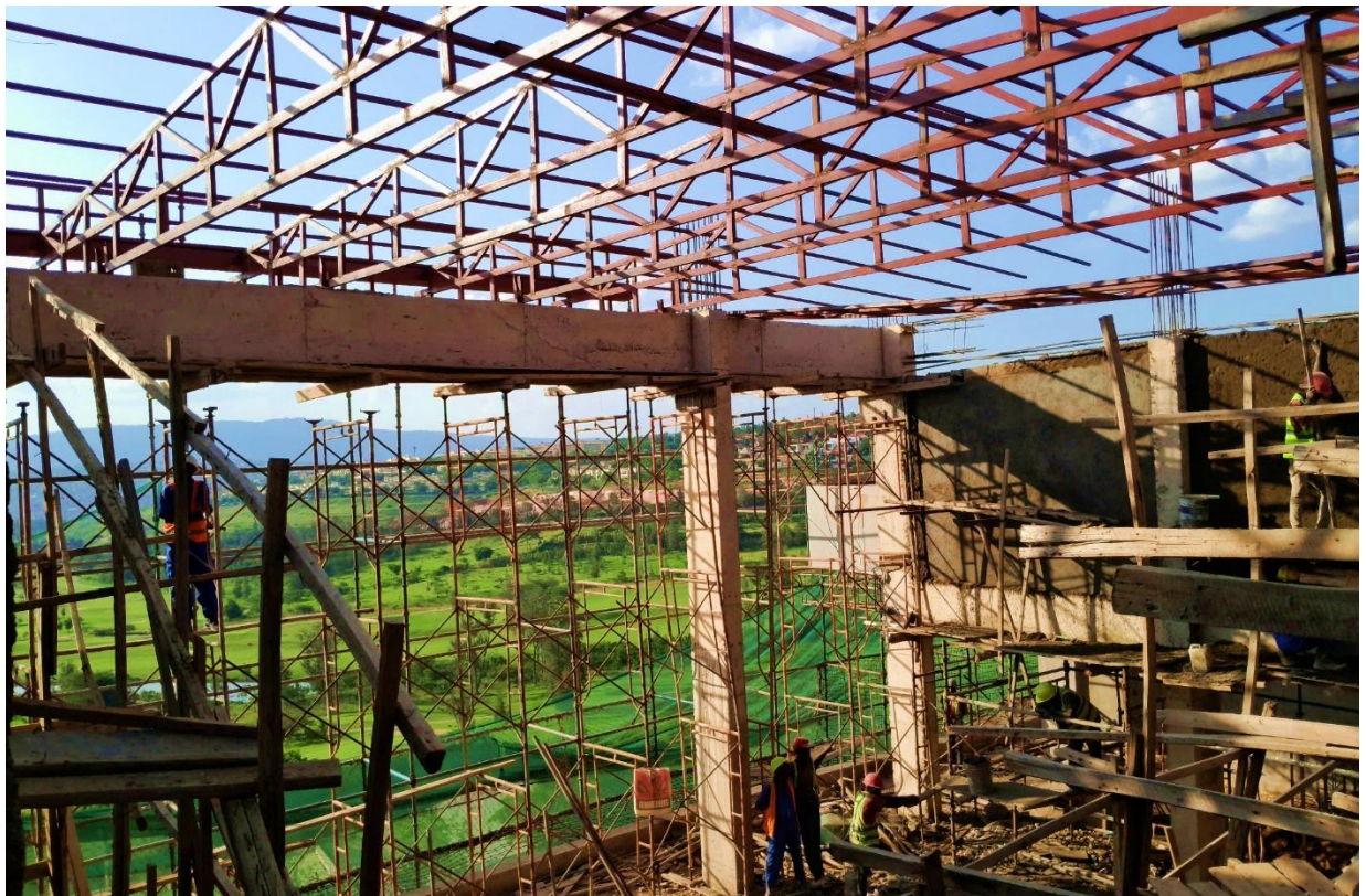
Phase 2 works showing: Roof truss installed in Lv. 2 of penthouse
