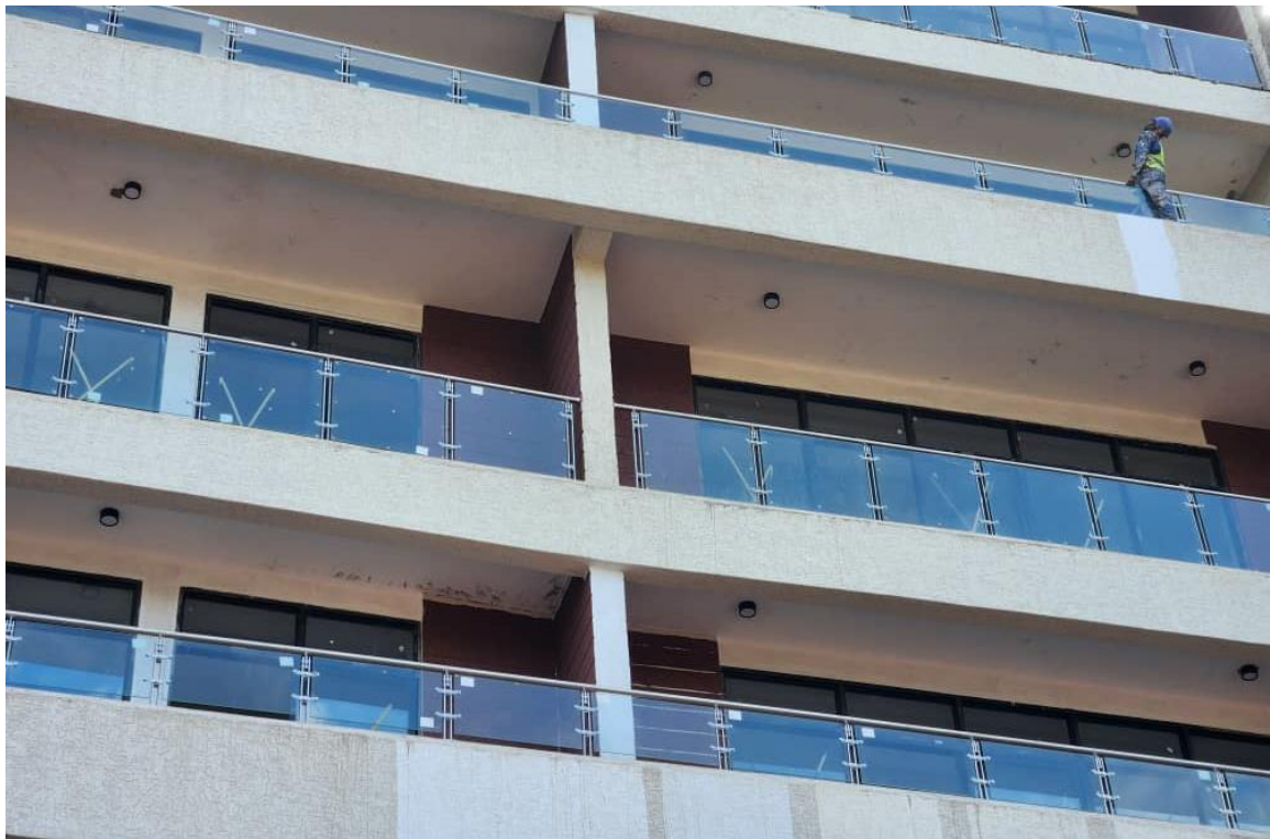
Phase 1, showing the painting works
