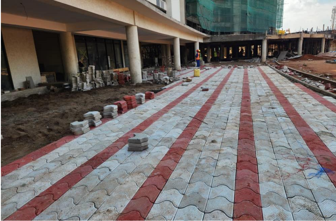
Phase 1 works paving works ongoing
