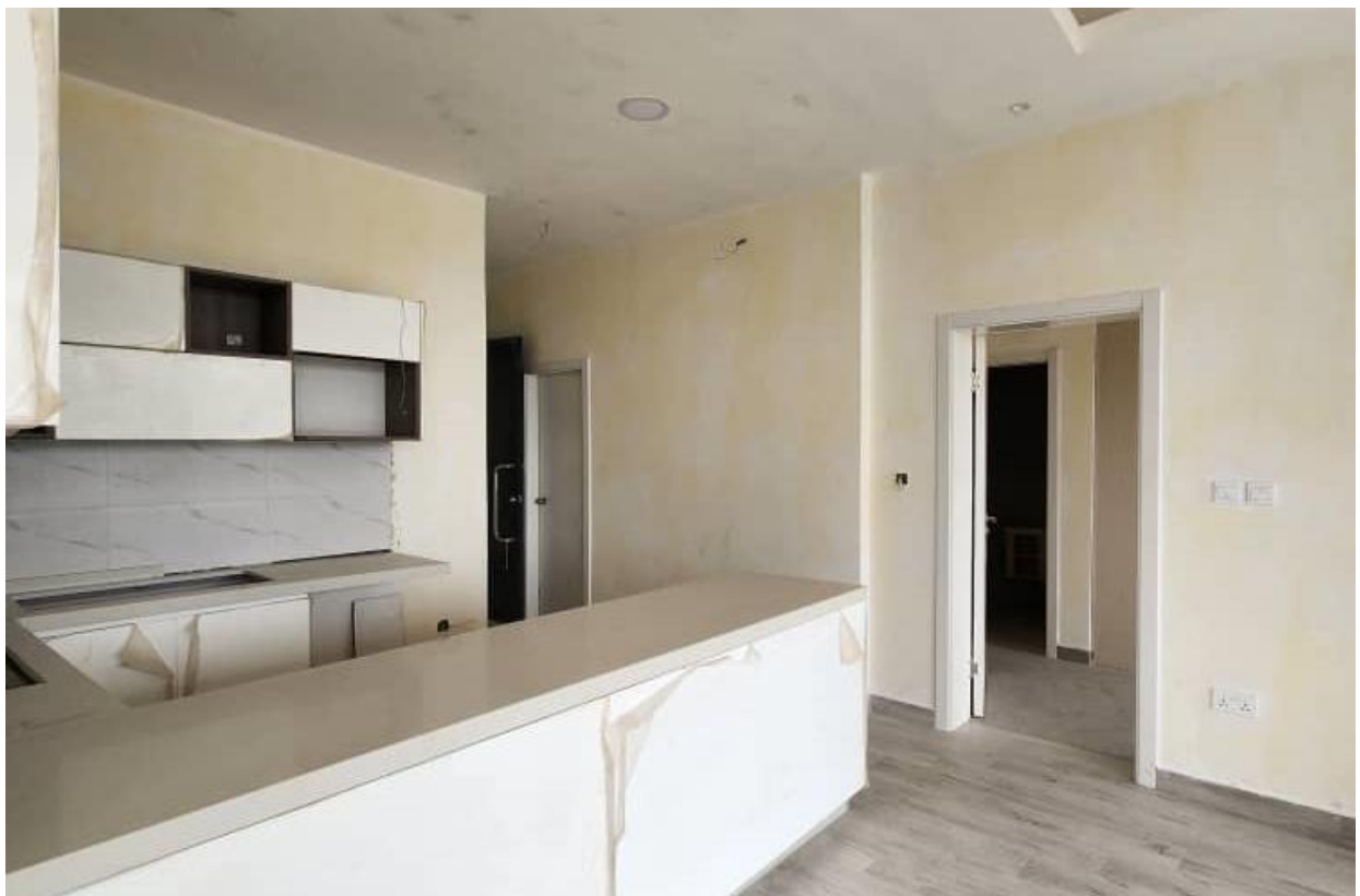
Phase 1, showing final painting works undercoat ongoing
