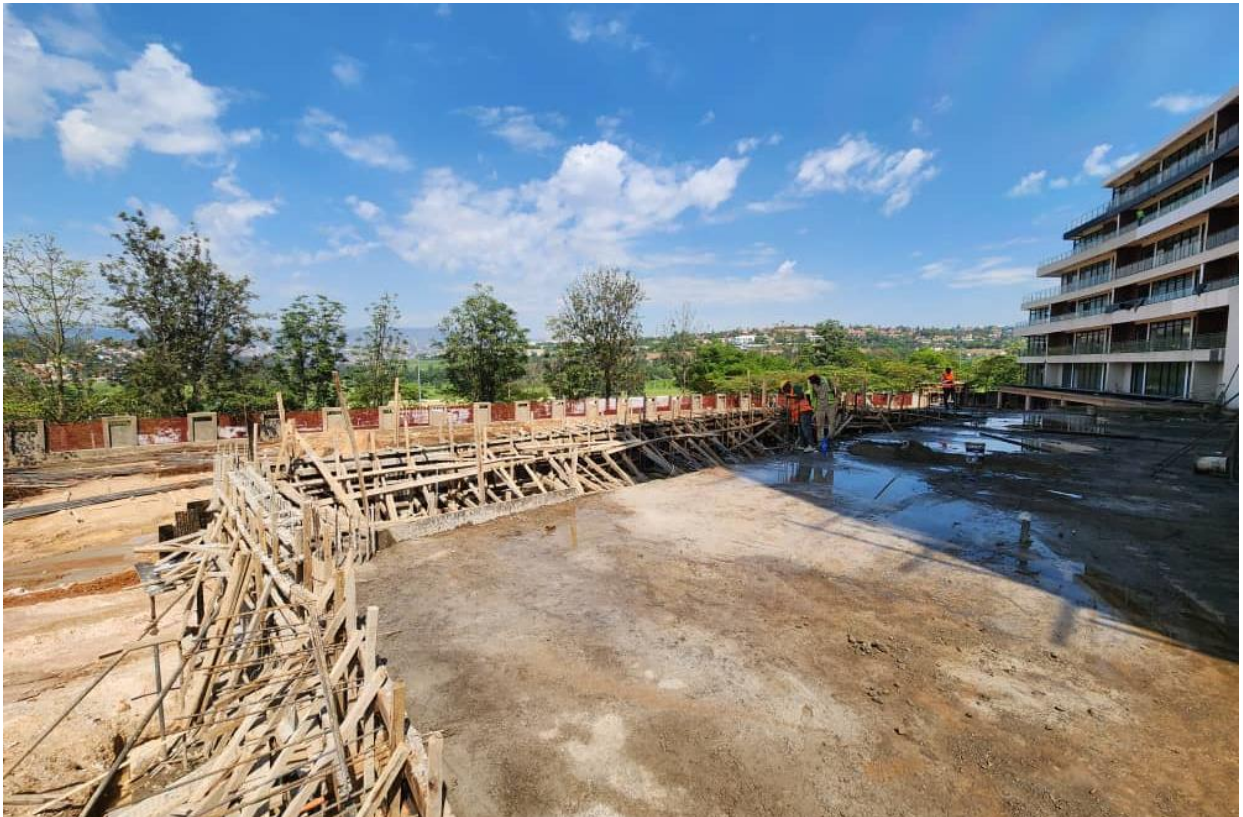
Phase 2 showing the pool deck and pool in the background
