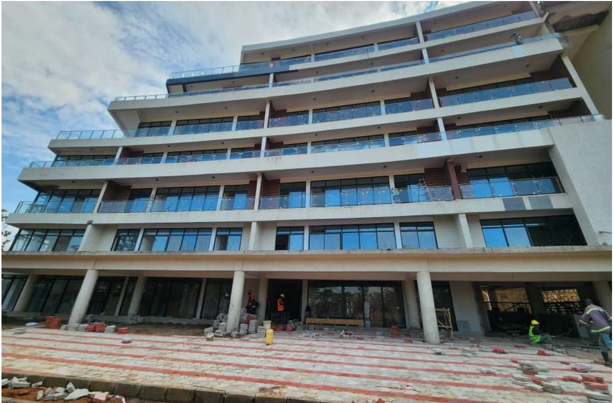
View of Phase 1, with paving and painting ongoing
