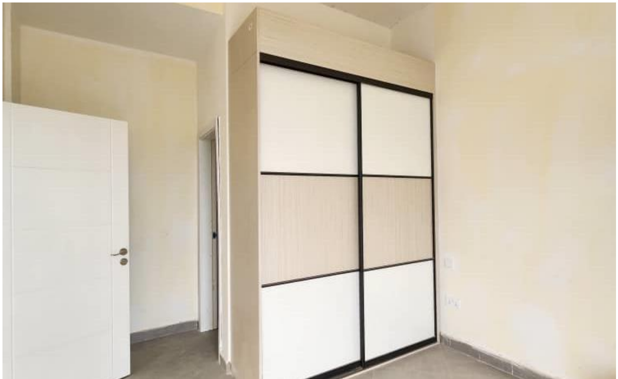
Phase 1 works showing: One of the bedrooms, with closets and doors
