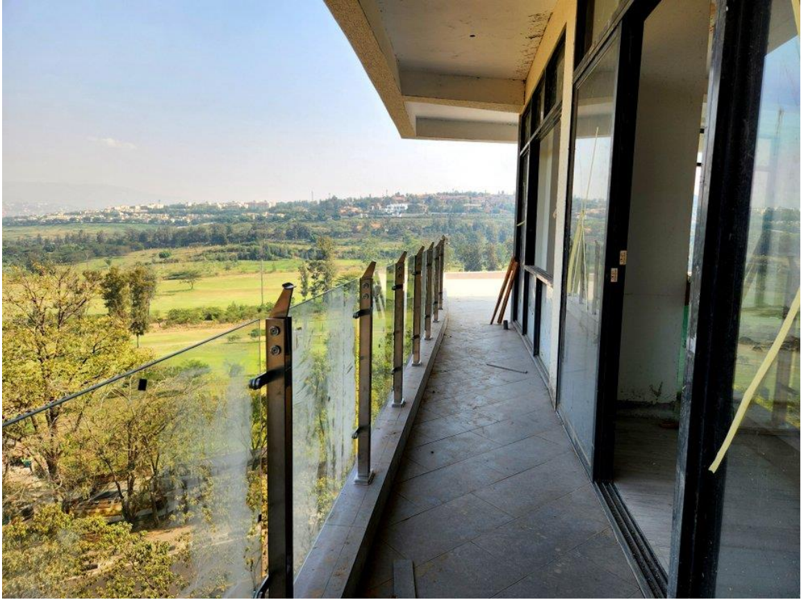
Glass balustrade installations ongoing
