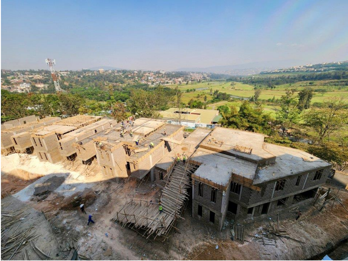
Townhouse construction progress
