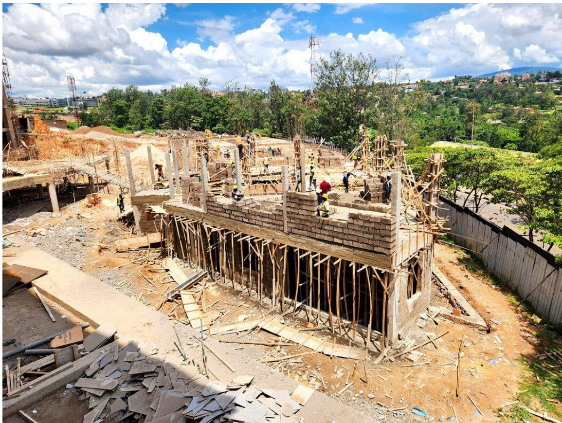
Townhouses construction ongoing
