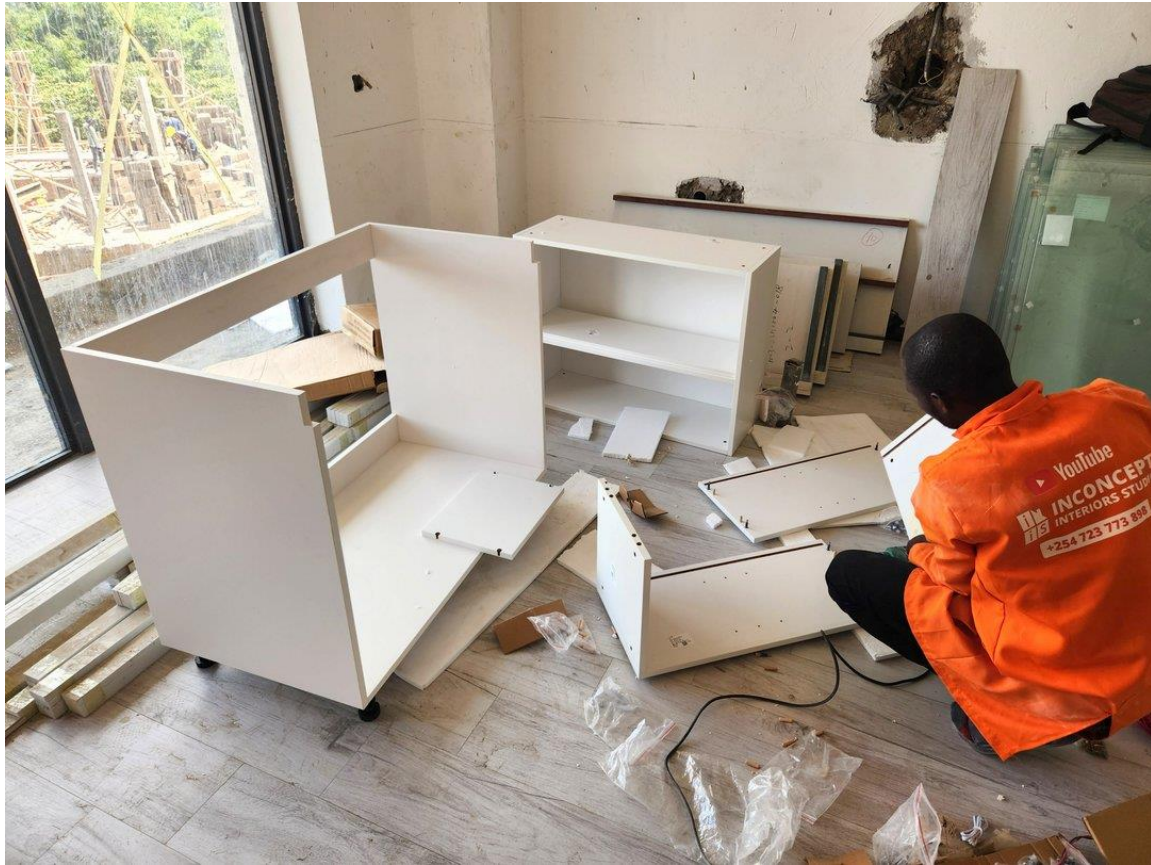
Kitchen professionals assembling the kitchen cabinets in phase 1
