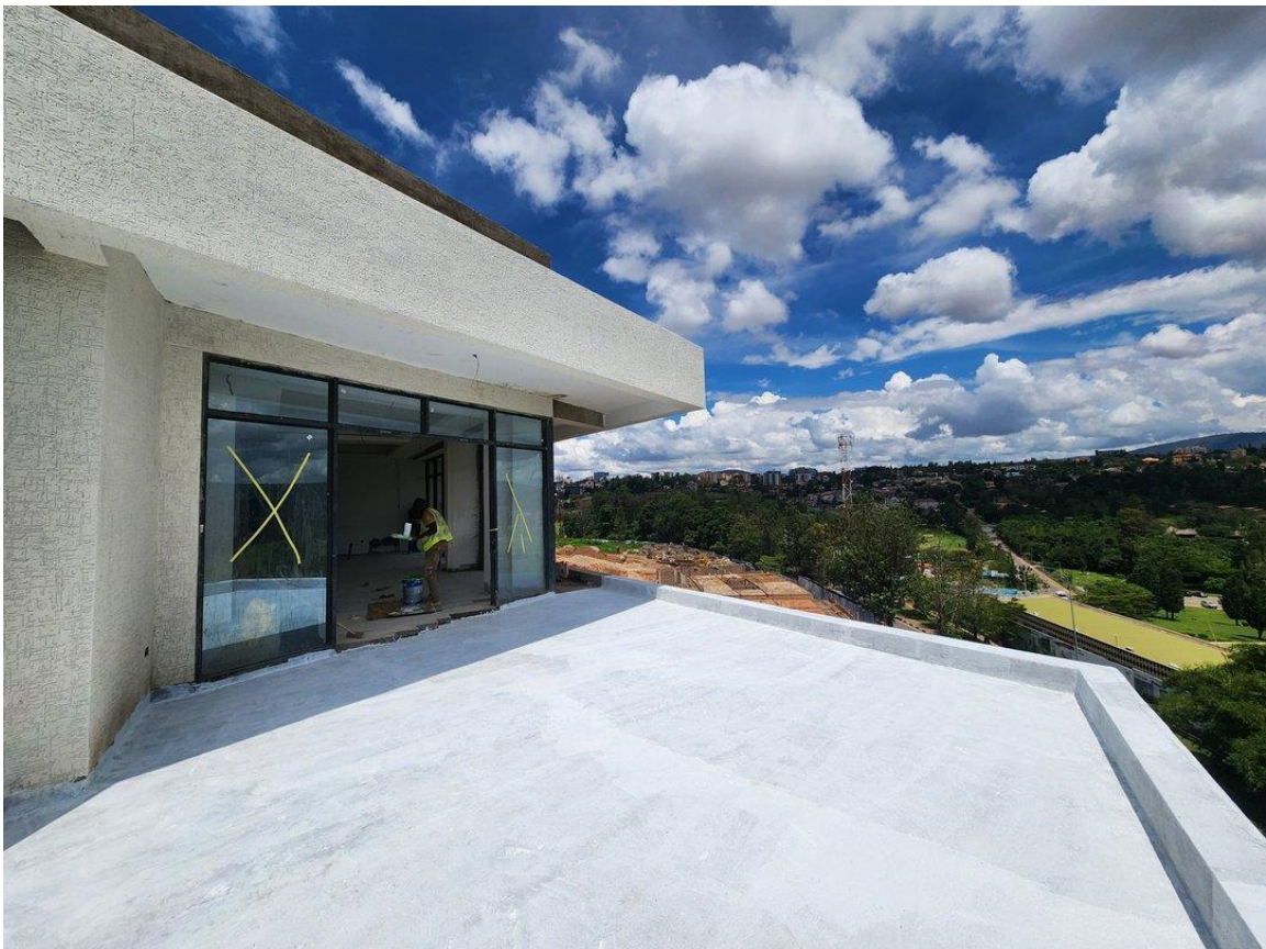
View from one of the terrace apartments at phase 1
