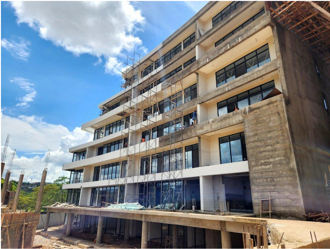
View of Phase 1 from the front terrace
