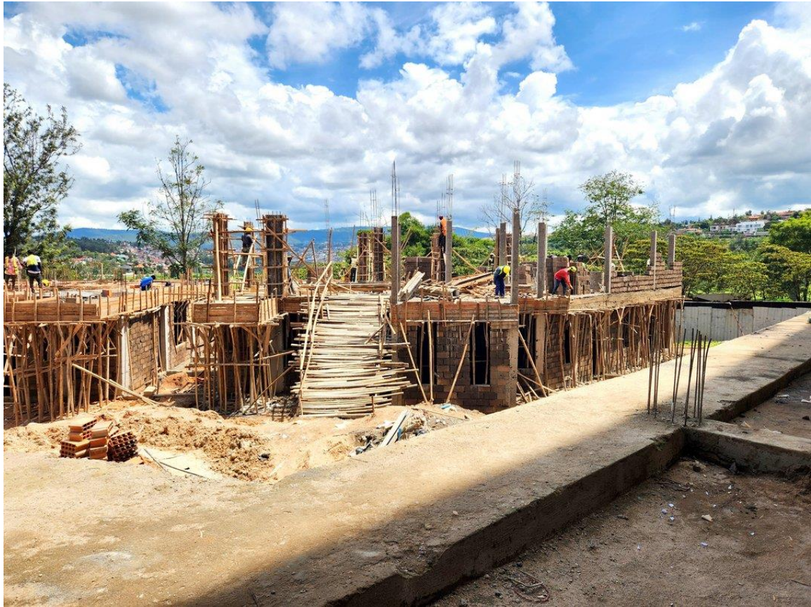
Townhouses construction seen from the terrace of phase 1
