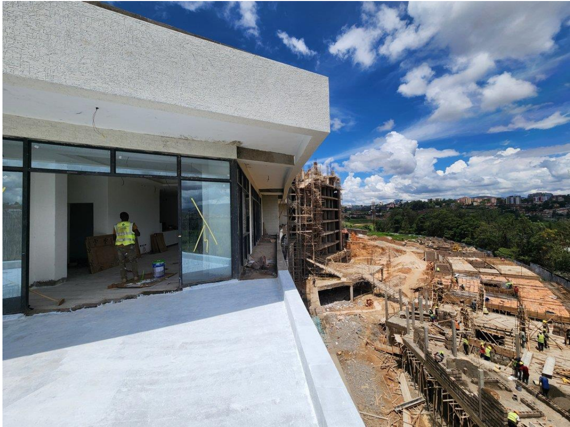
Townhouse progress seen from a terrace apartment at phase 1
