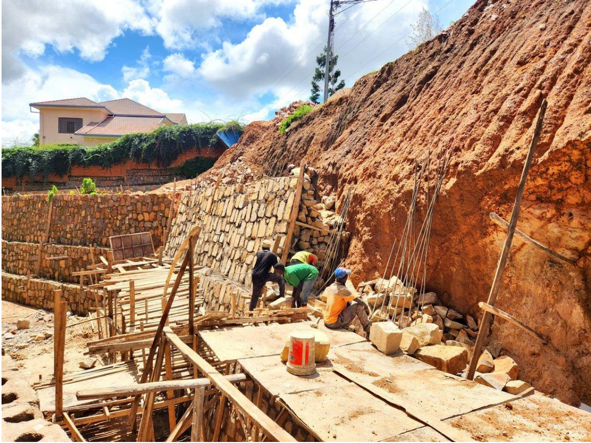
Retaining wall construction in phase 2
