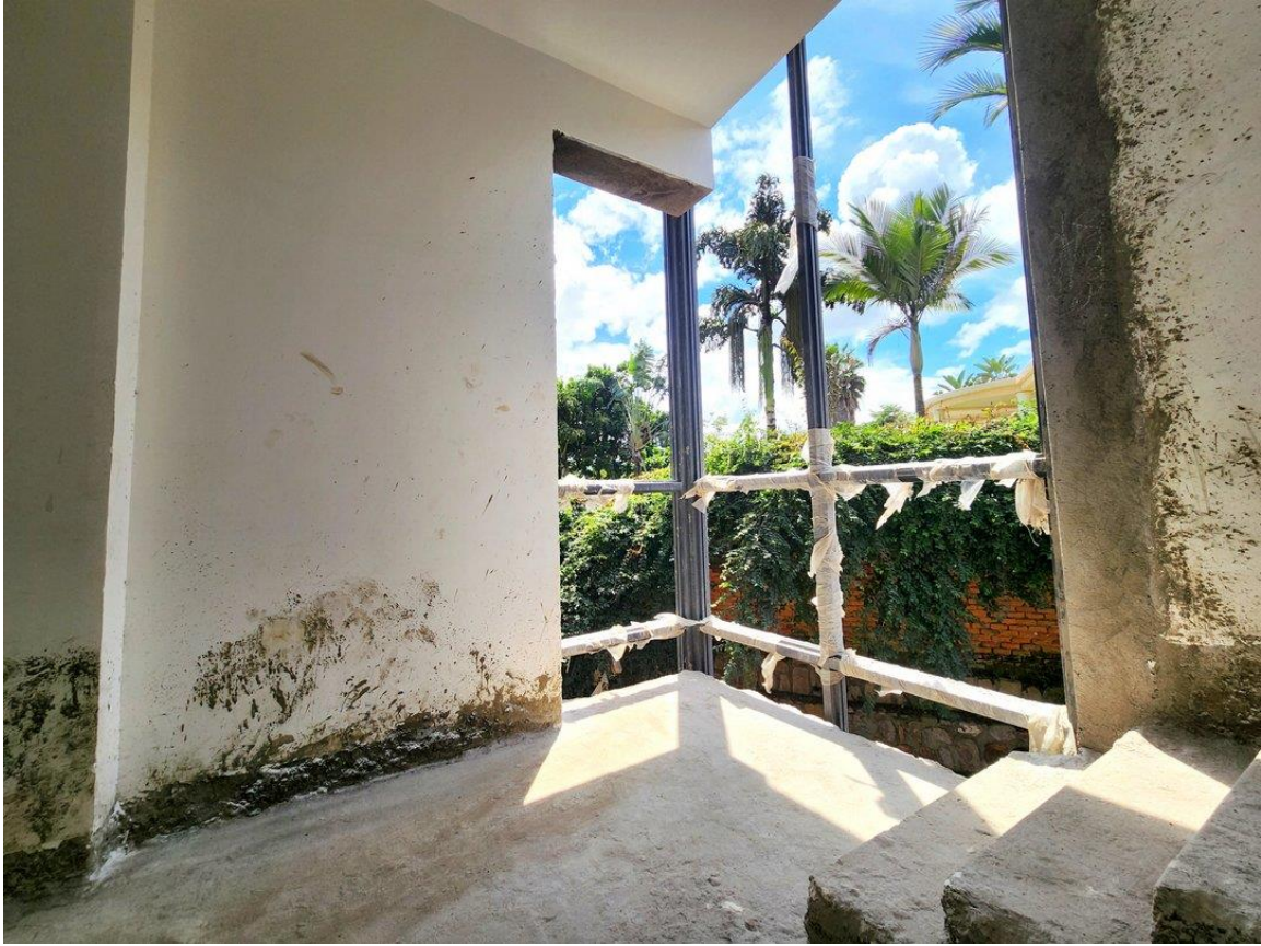
Landing area aluminum glass works ongoing
