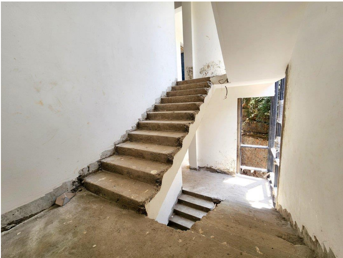
Staircase in phase 1
