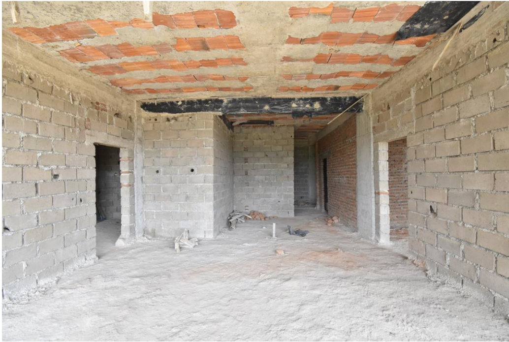
Phase 2 apartments taking shape
