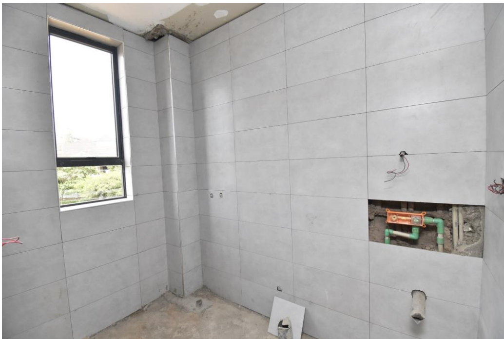
Bathroom works ongoing at Phase 1
