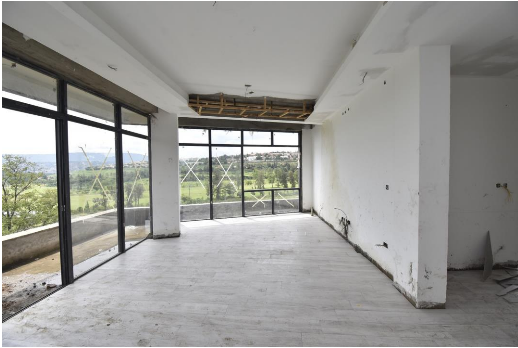
One of the side units at Phase 1
