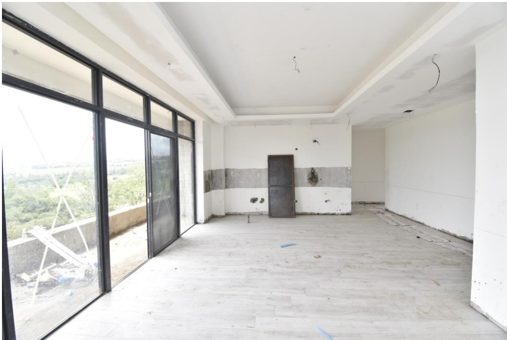
One of the units, showing the kitchen in the background, Phase 1
