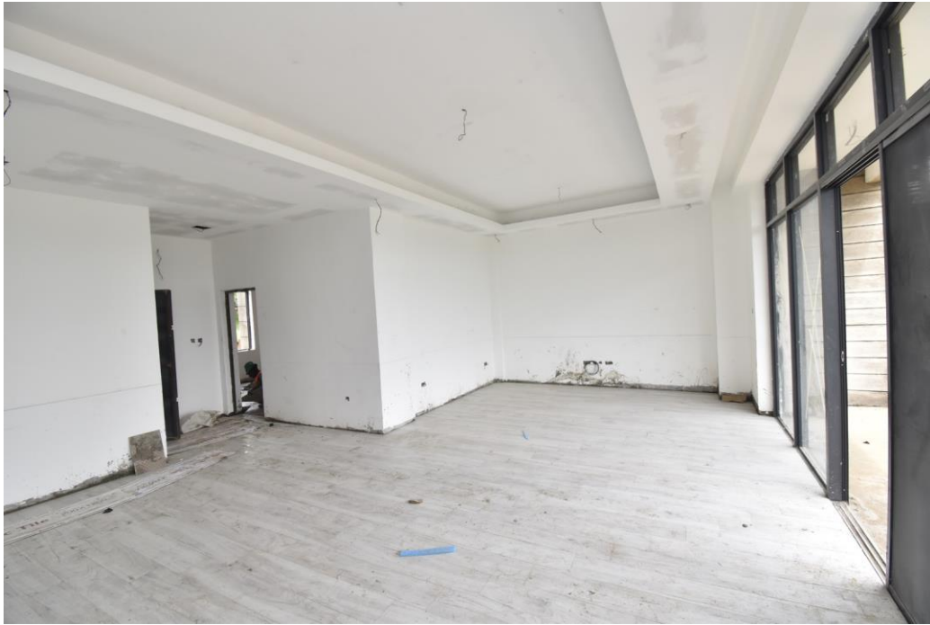
Finishing works for Phase 1 ongoing
