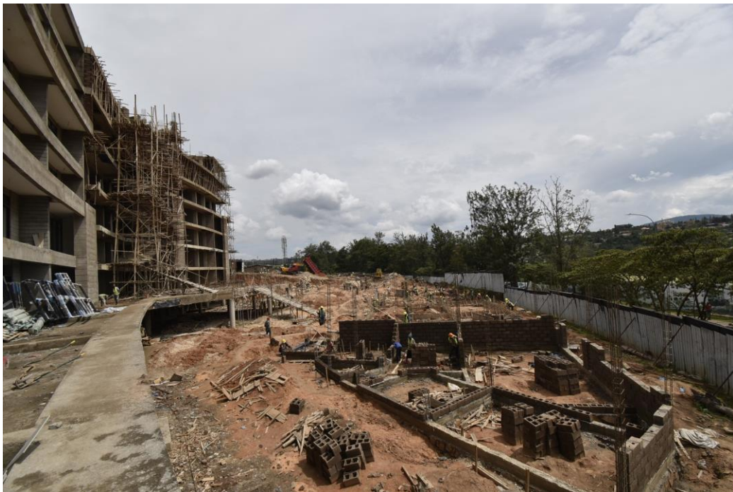
Townhouses construction ongoing
