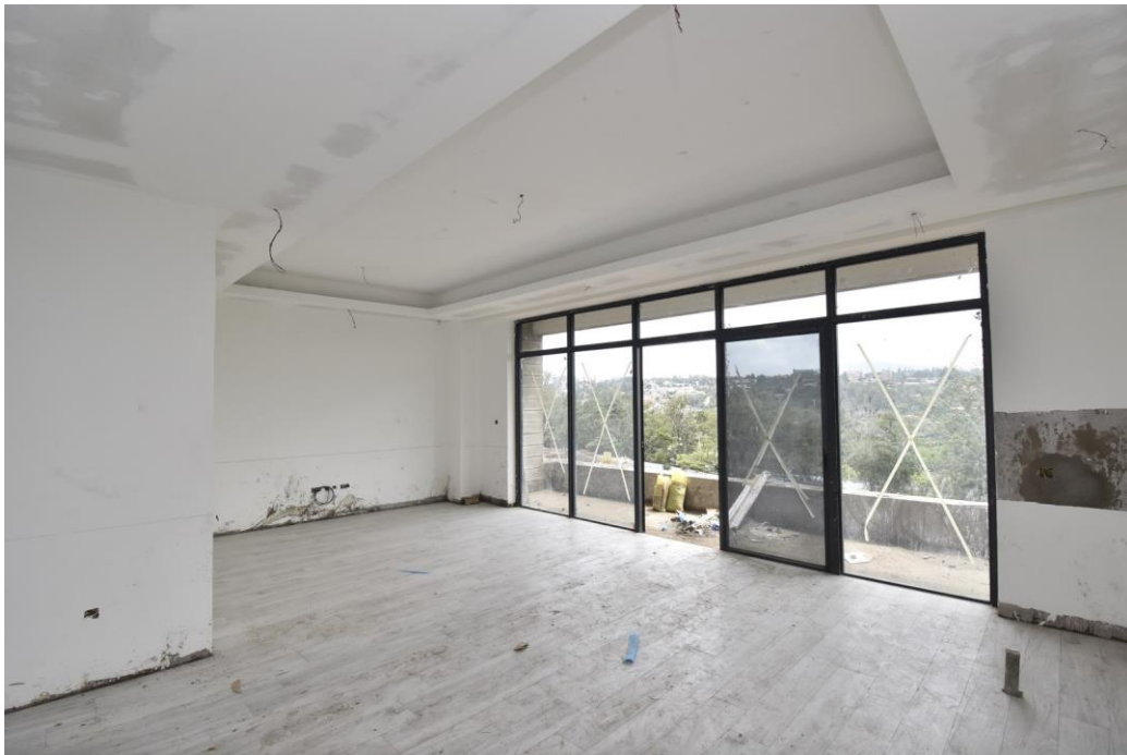
Living area in one of the Phase 1 units
