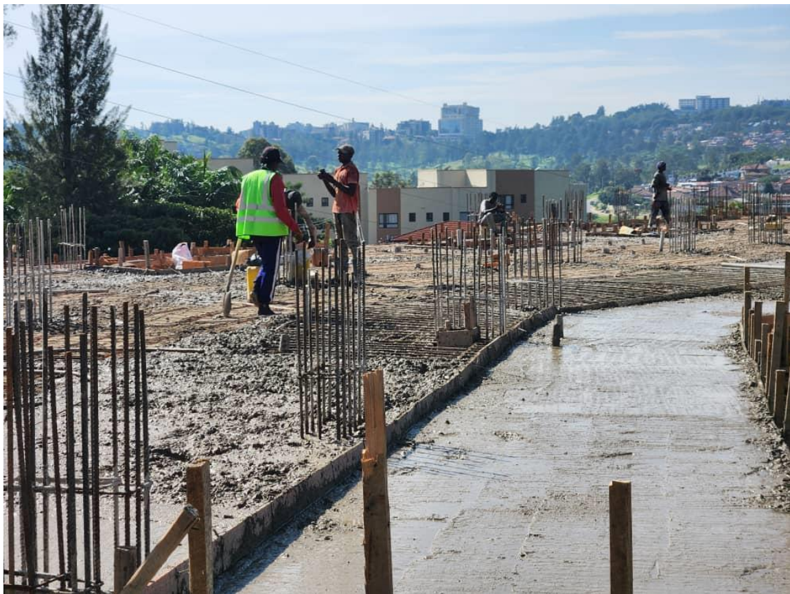
4 th Floor, Phase 2 slab casting
