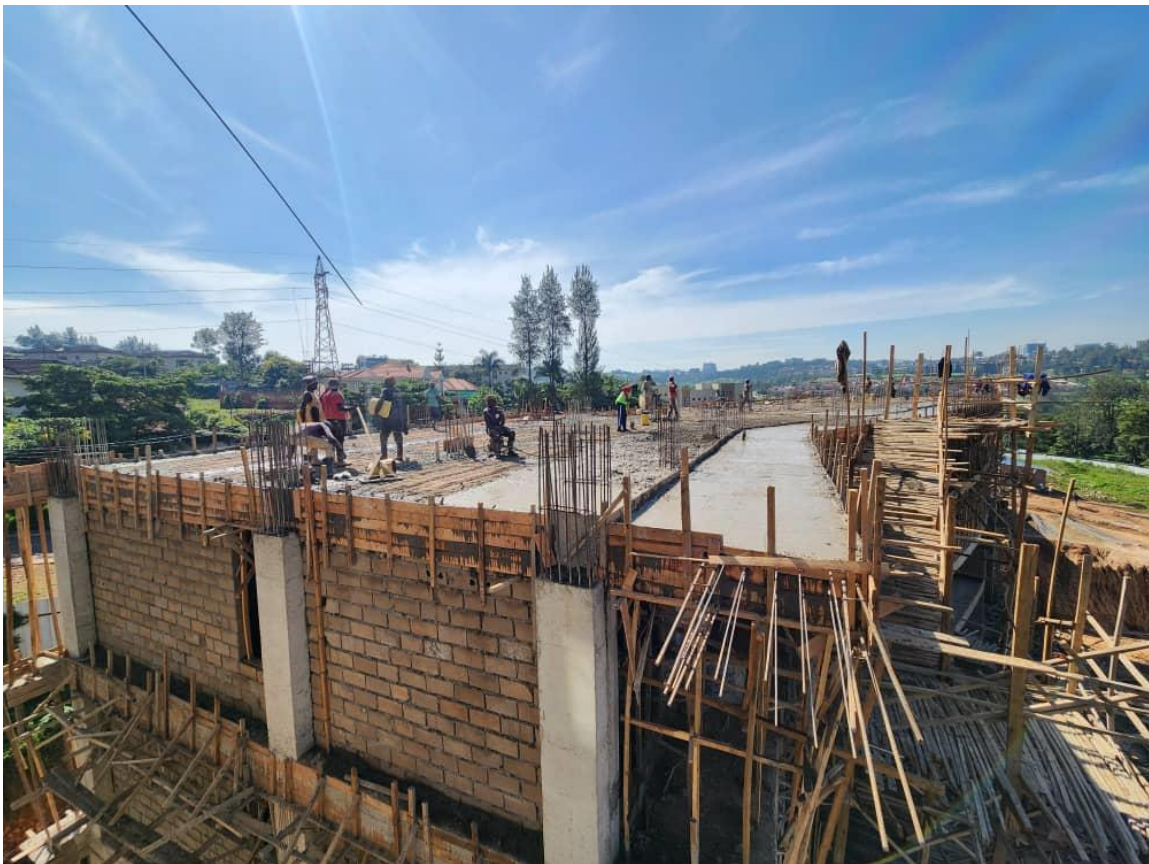
Phase 2 progress as seen from Phase 1
