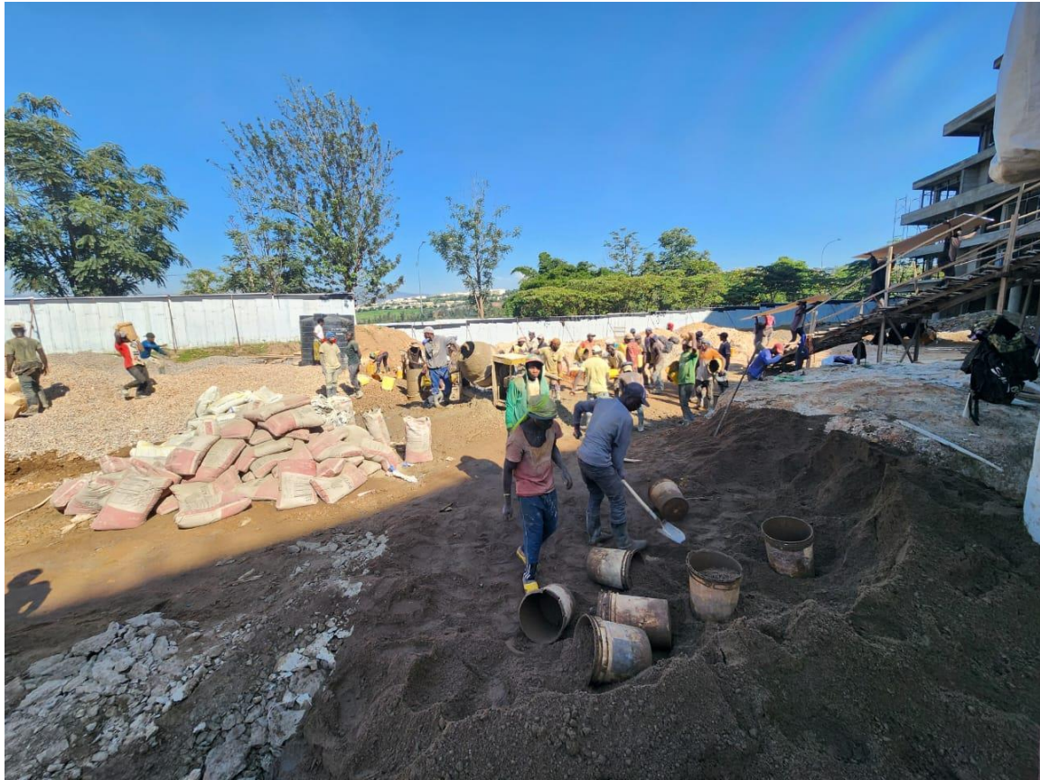
Men at work on concrete mixing and slab casting, Phase 2
