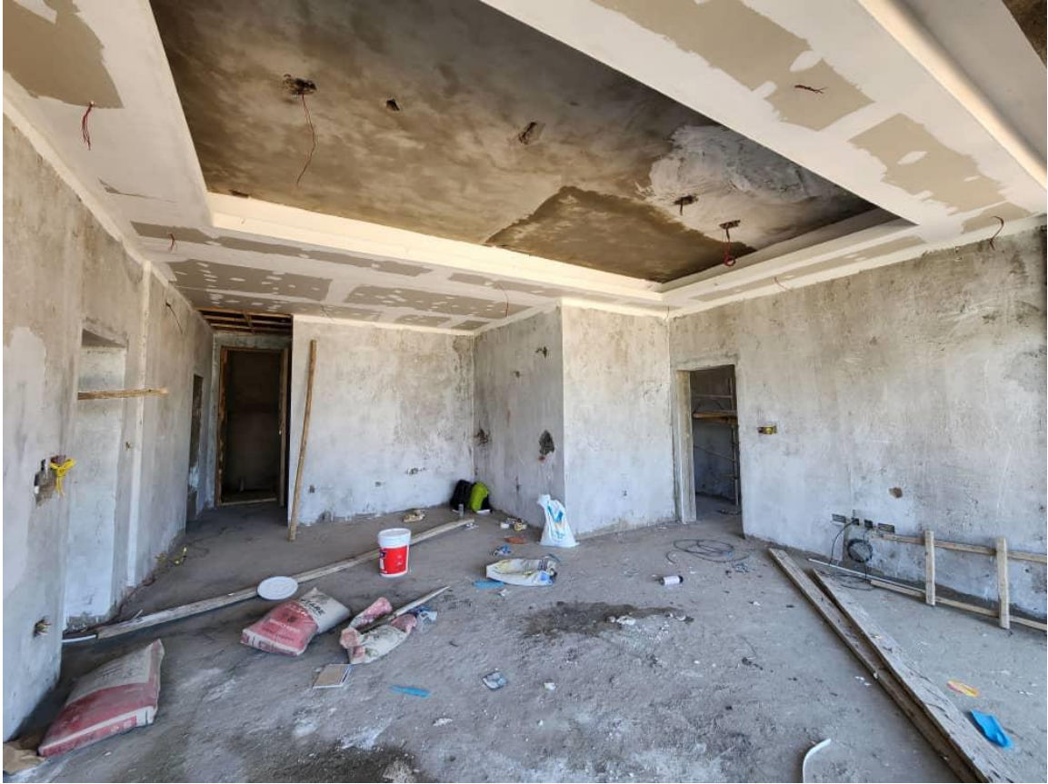
Phase 1 gypsum works and initial painting
