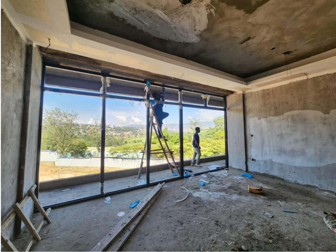
Curtain wall fixing and installation.
