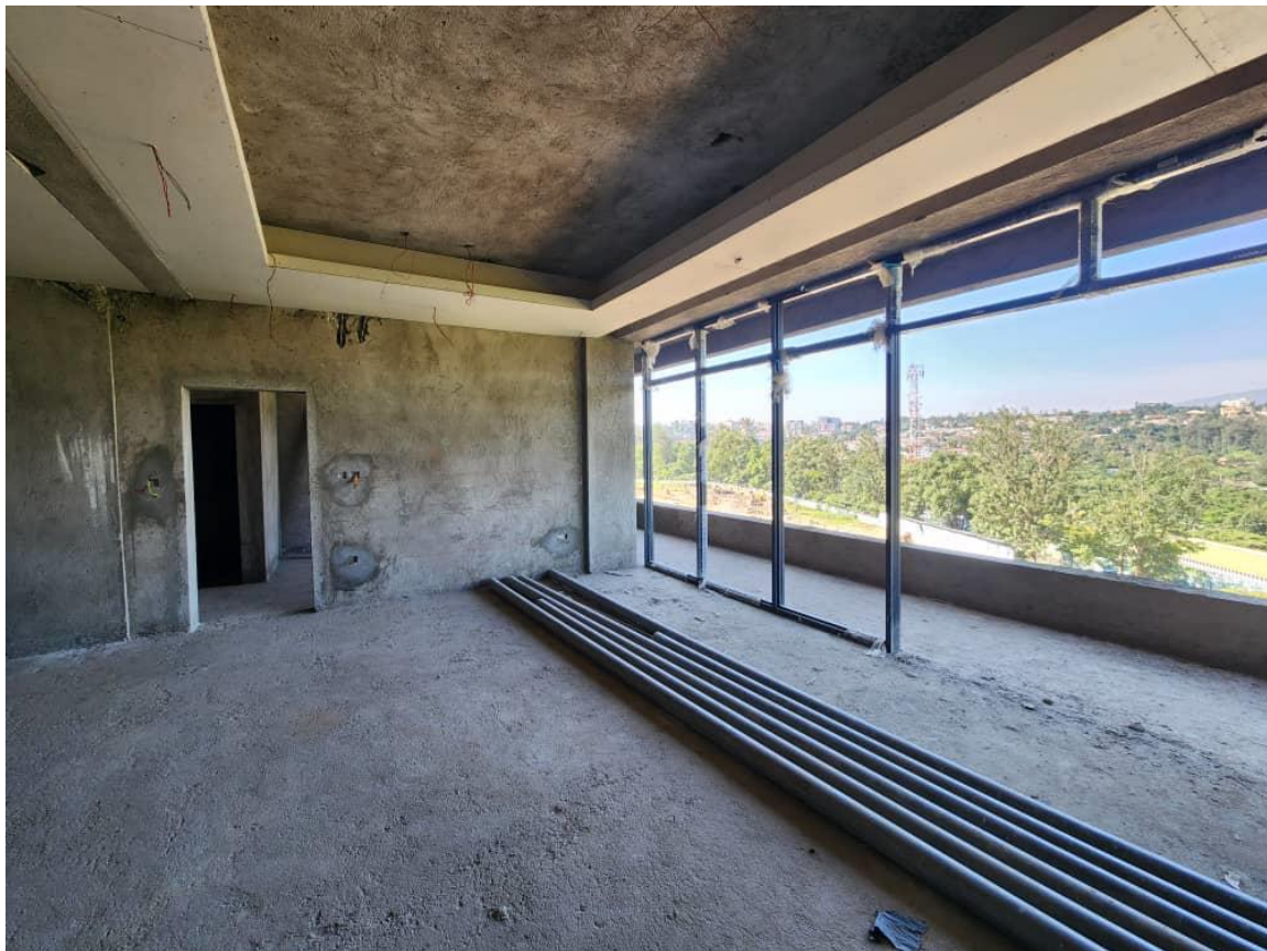
Gypsum board works on going
