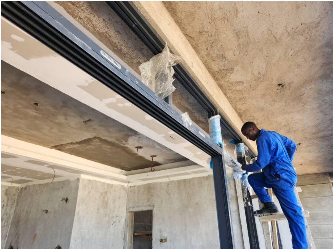
Curtain wall installation progressing well at Phase 1
