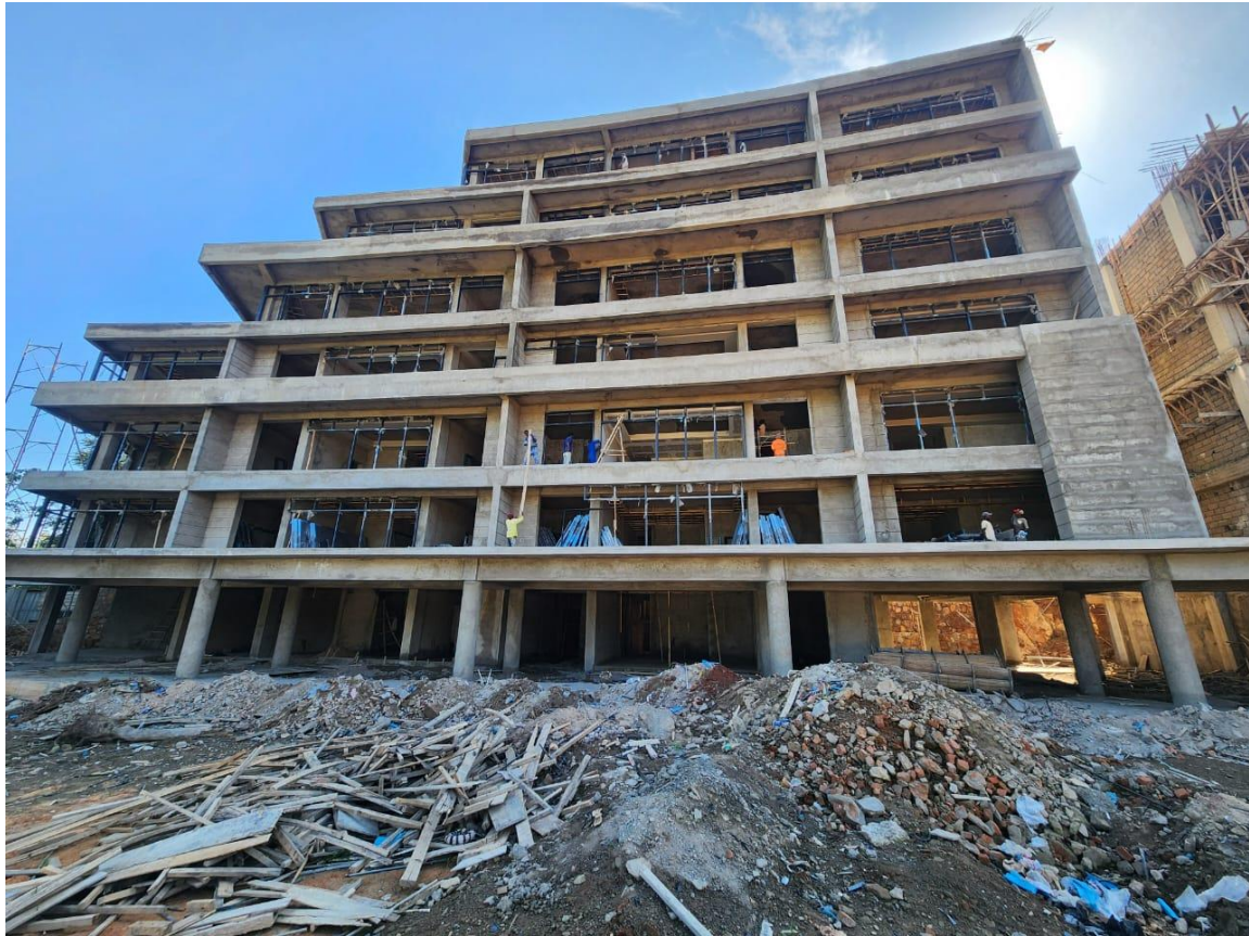
Front View of Phase 1
