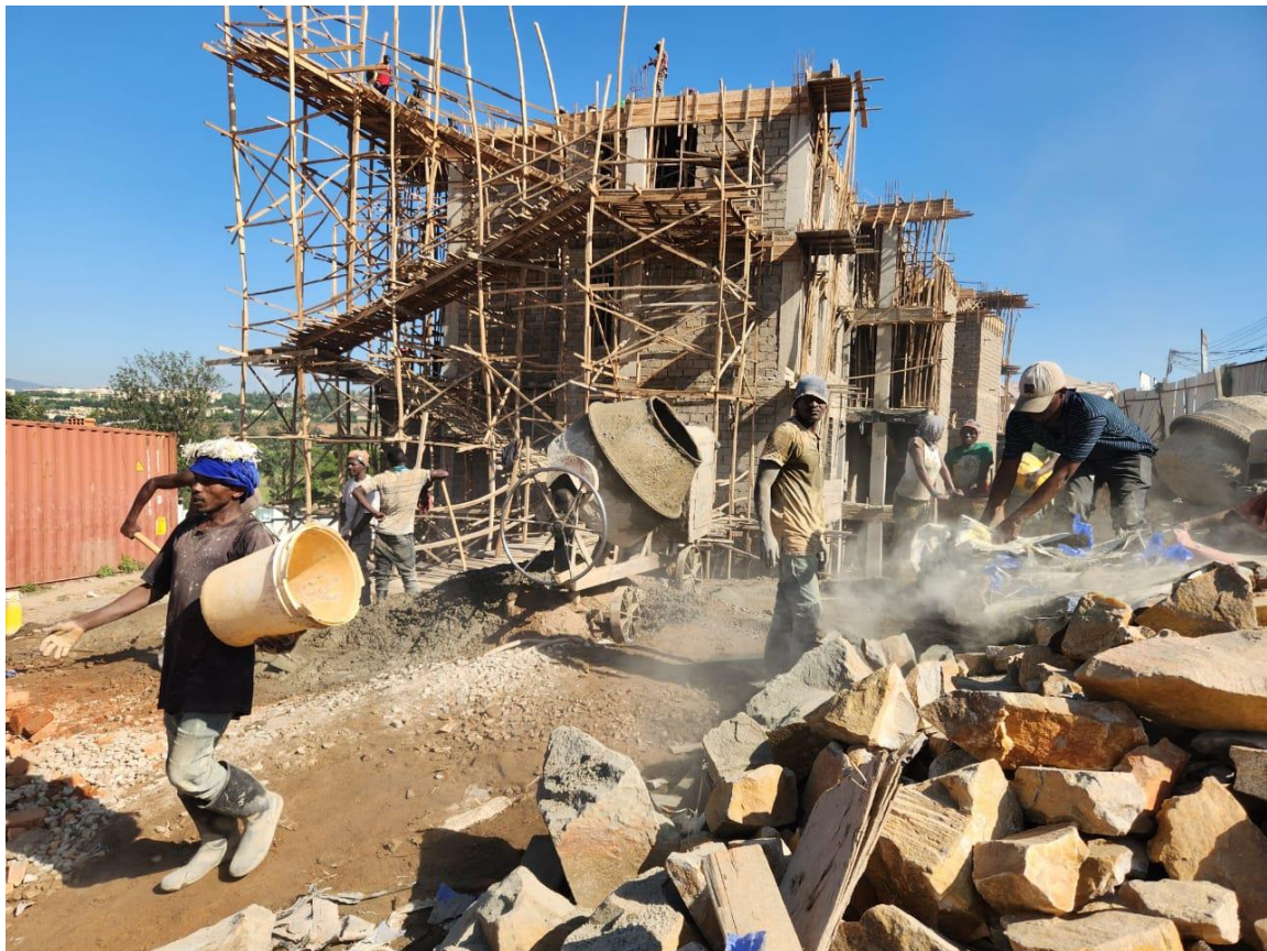
Mixing Concrete for slab casting at Phase 2
