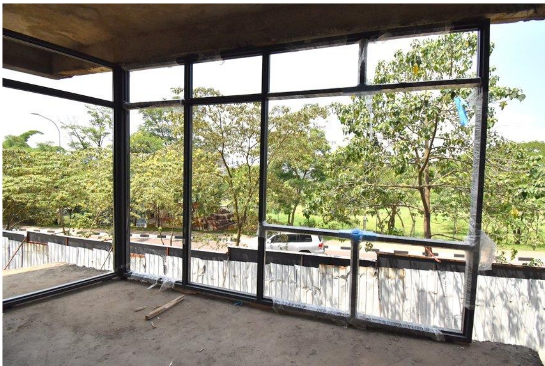
Curtain wall fixes ongoing at Phase 1
