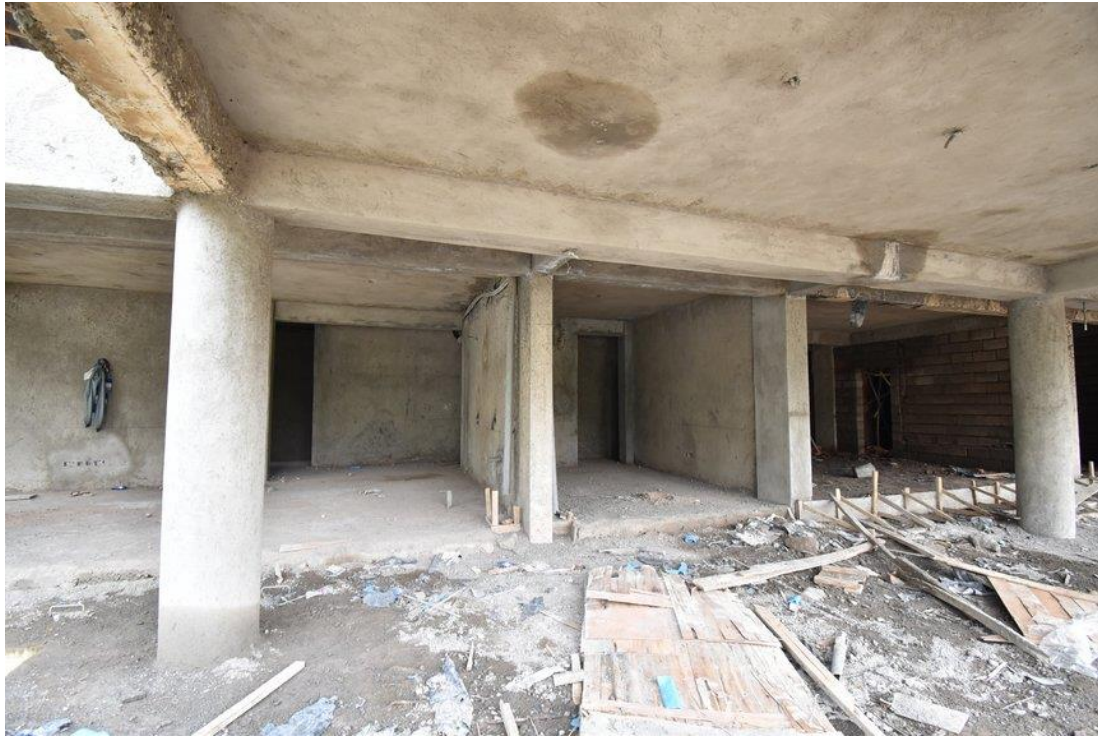
The basement at Phase 1
