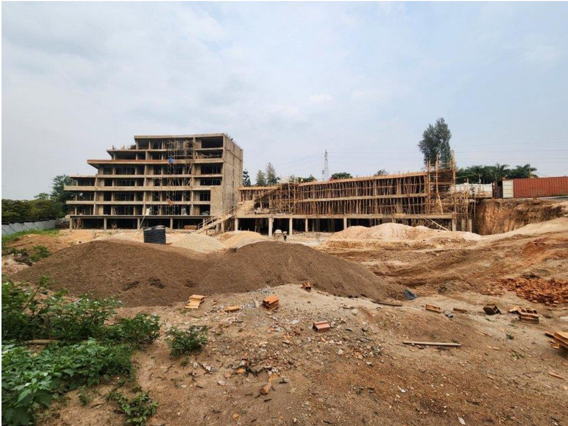
Phase 1 and 2 seen from the front
