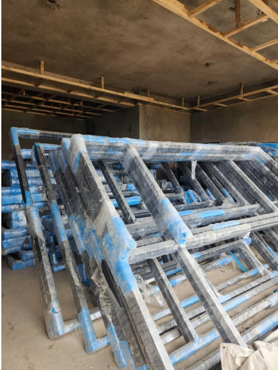
Aluminium doors windows at site
