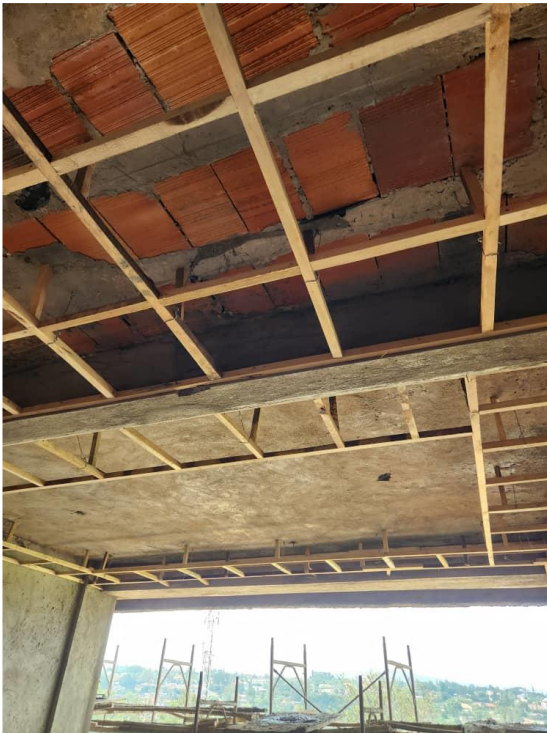
Gypsum ceiling works
