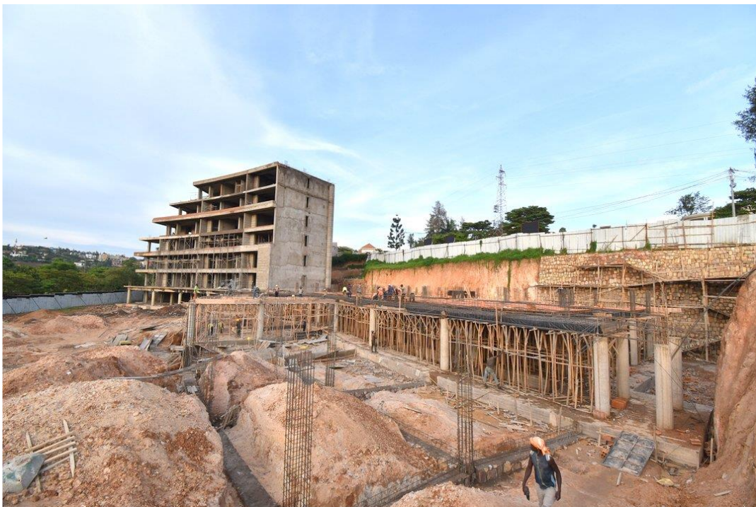
Phase 2 works ongoing
