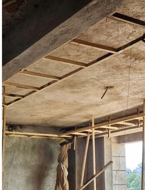
Gypsum ceiling preparations
