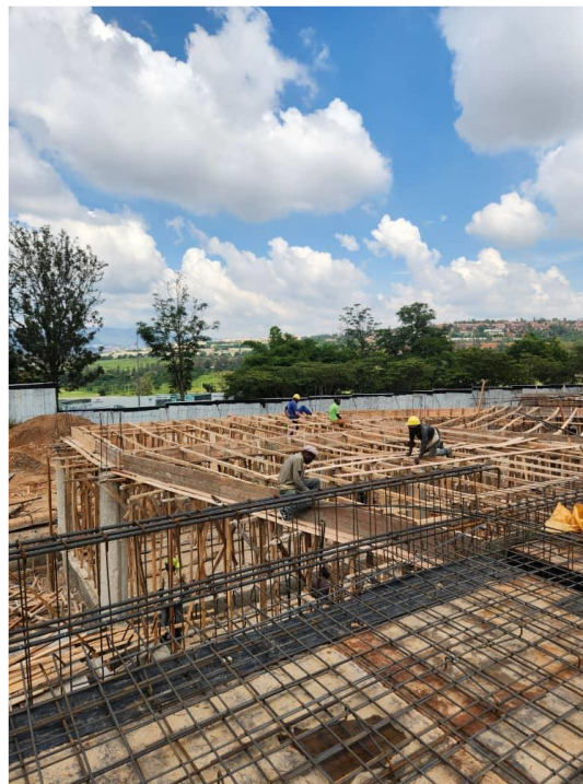
Phase 2 terraces works
