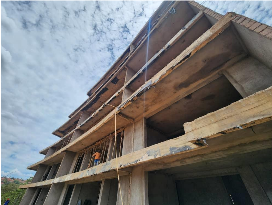
View from the ground floor
