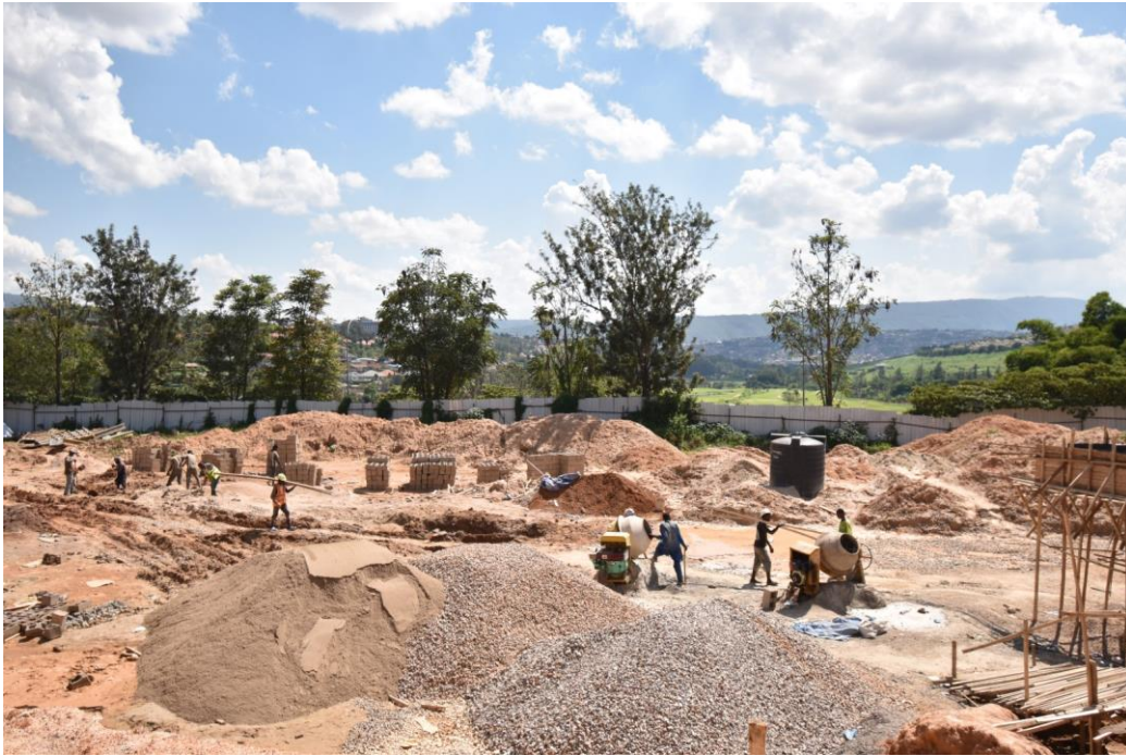
Concrete mixing ongoing at the site
